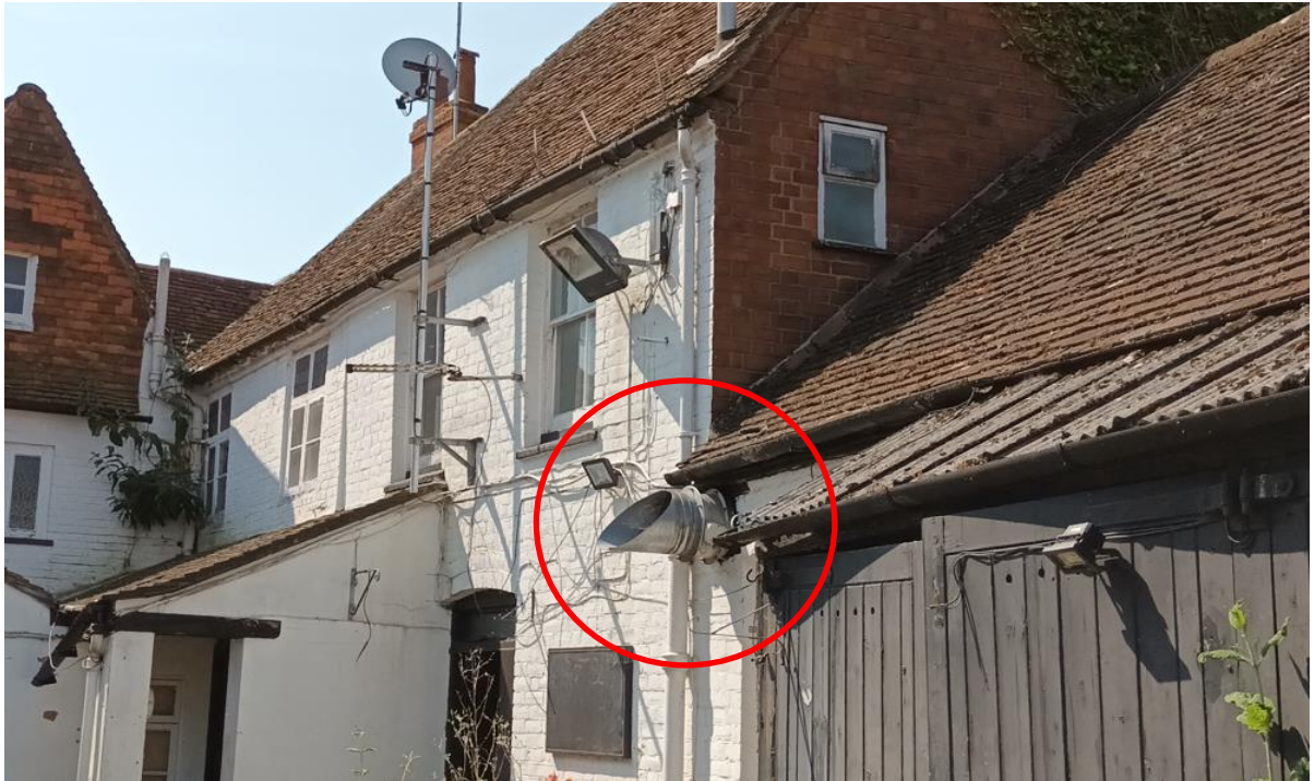
Figure 2: Existing kitchen extract position
