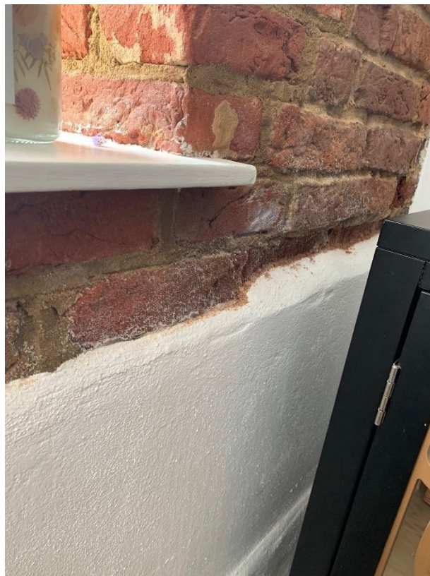
Figure 3 Salting above render close up
