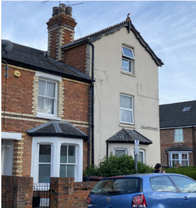
Figure 6 no 114 Queens Road corner plot scale
