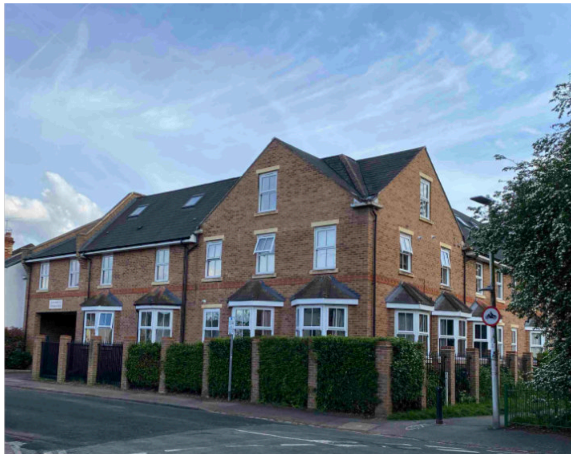
Figure 14 Flatted development, no 129 Queens Road
