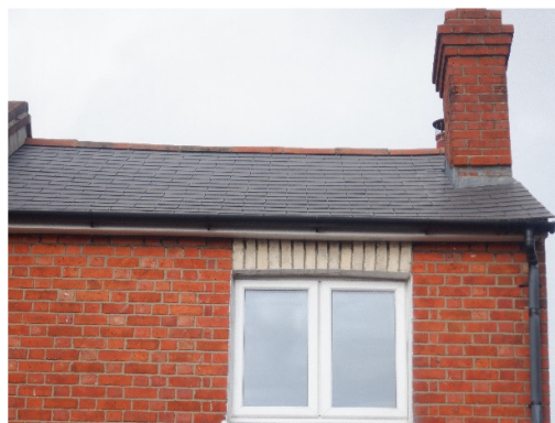
4. Ridge mortar intact throughout.
