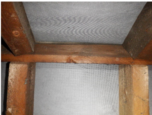
17. Breathable roof membrane liner throughout.
