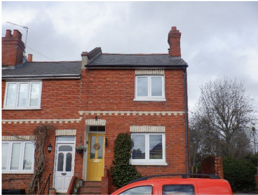
1. Front of property viewed from south.
