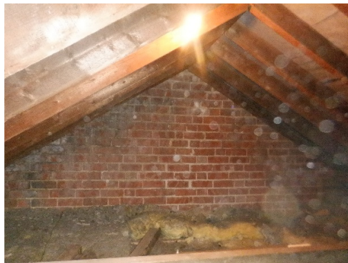
12. Brickwork gable end party wall (western).
