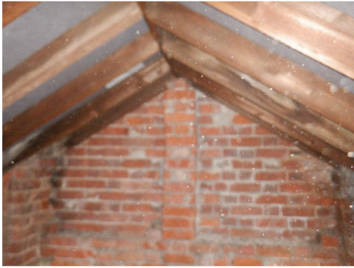
13. Brickwork gable end (eastern).
