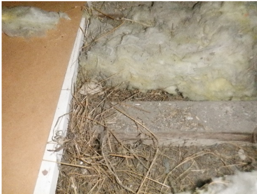
21. Straw visible under insulation.
