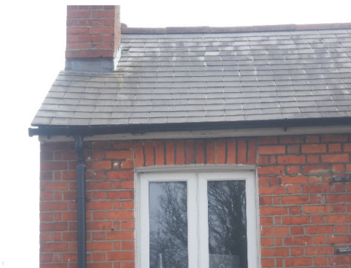
3. Tight flat slate roof tiles throughout.
