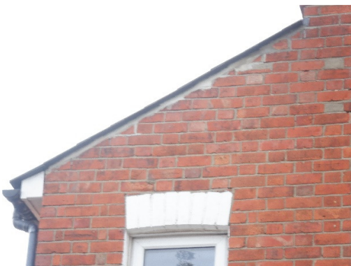
5. Gable verge mortar mostly intact
