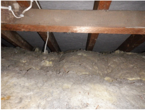
19. Fibreglass insulation up to eaves.
