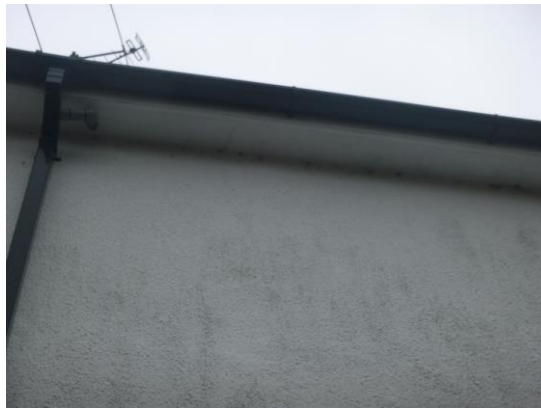
8. Fully sealed soffits at eaves (northwest elevation).
