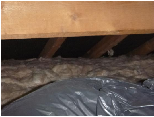
13. Fibreglass floor insulation (roof void).
