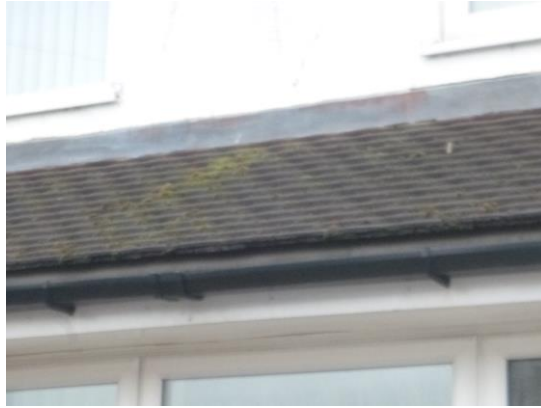
4. Flat overlapping roof tiles on front porch (front elevation).
