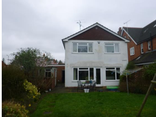
2. Rear of house viewed from southwest.
