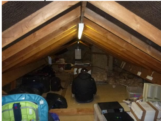
10. Roof void viewed from front gable end.
