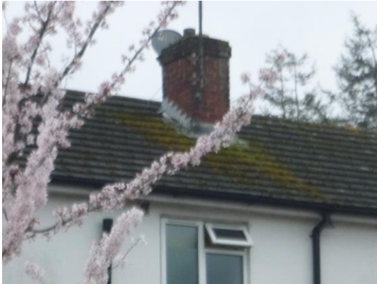
3. Large, interlocking concrete roof tiles (northwest elevation).
