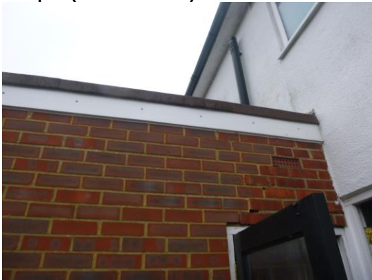
9. Bituminous flat roof and tight uPVC fascia on attached garage (rear elevation).
