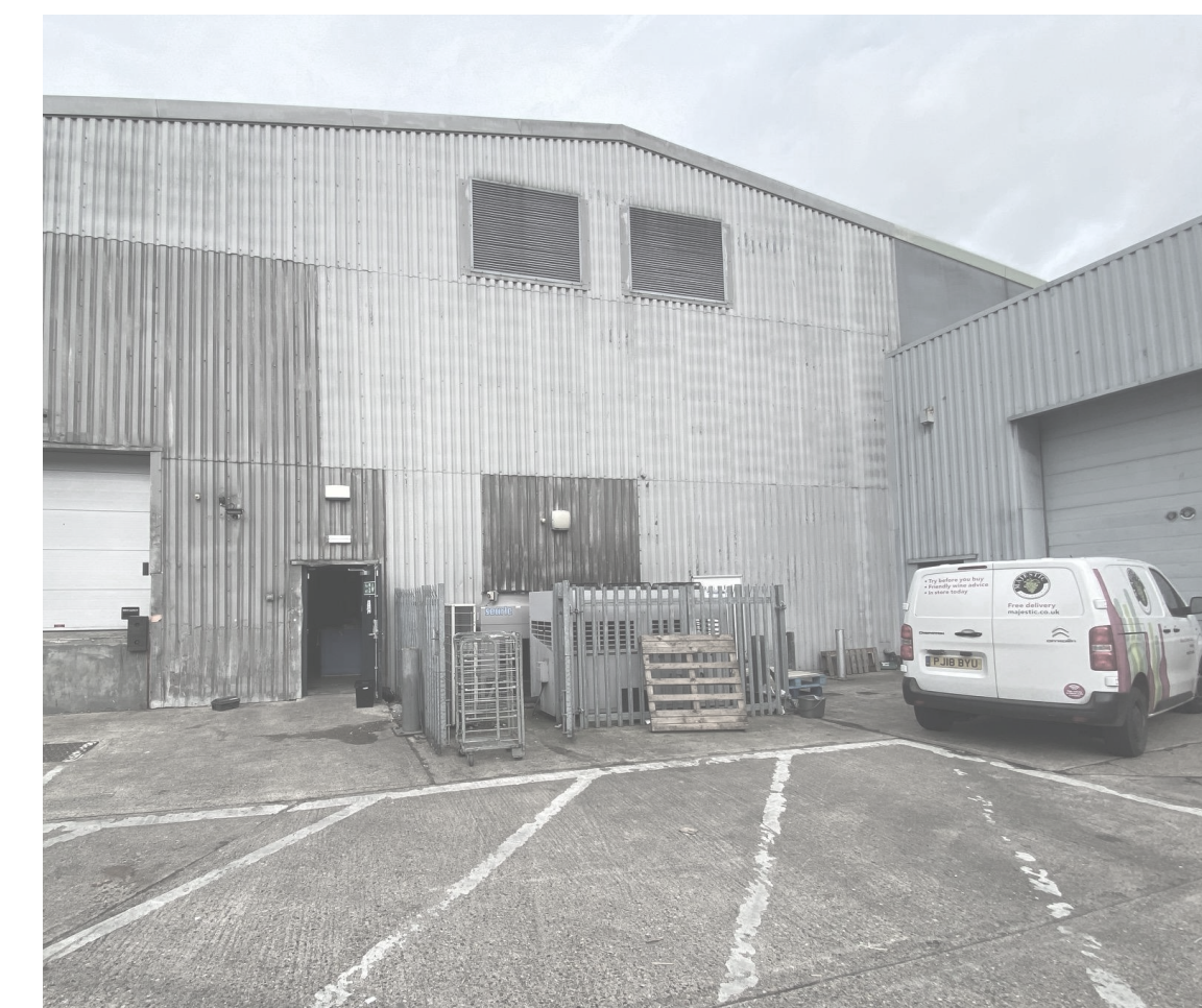
A View of existing plant compound from service yard
