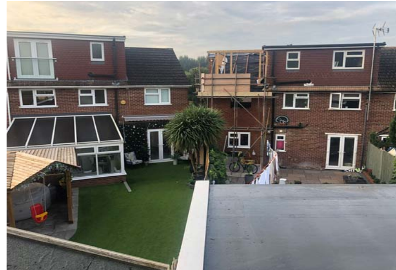
Rear of number 32 Ashampstead Road, Reading showing the framing of the later (and now removed) dormer window
