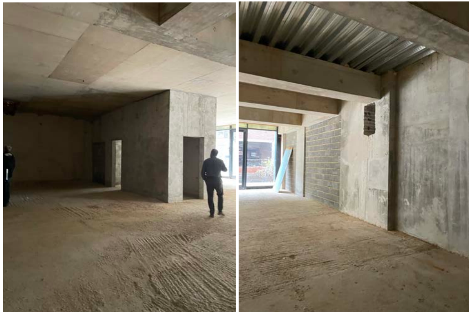
Photograph of the Lower Ground Floor and the hole for the flue to the roof
