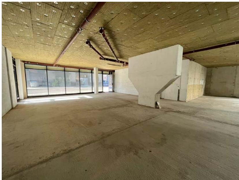
Photograph of the Ground Floor showing the acoustic separation between the ground and first floors completed to satisfy a planning condition.
