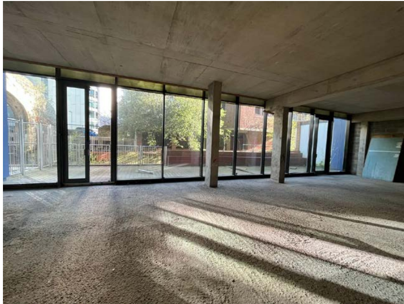
View across Lower Ground Floor towards Holy Brook.
