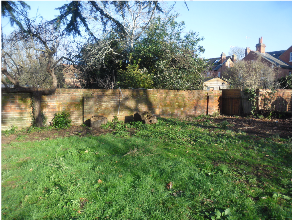
The boundary wall between nos. 39 and 41a Eastern Avenue
