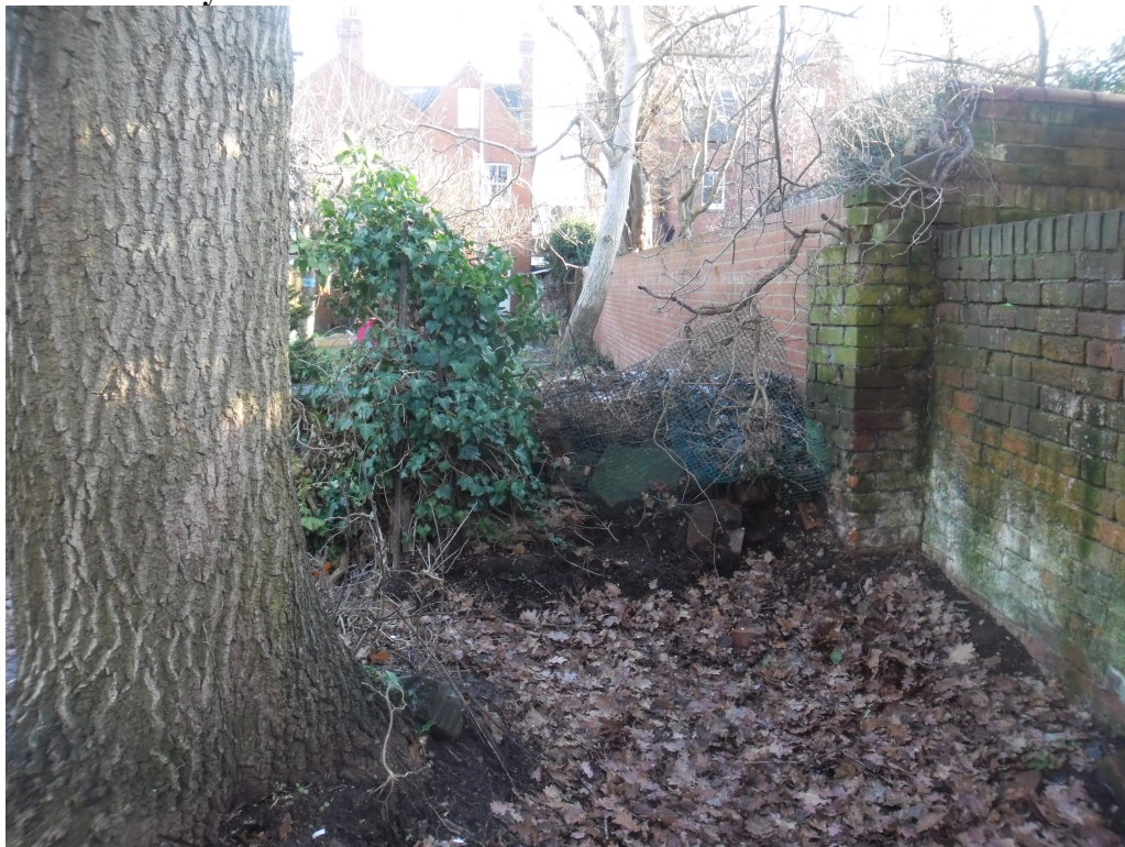
The boundary wall between nos. 86 and 88 Hamilton Road, Reading.
