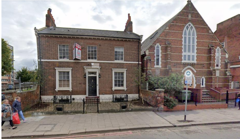
2.13 This shows the front together with the adjoining building, the Providence Chapel. The chapel is not listed.
