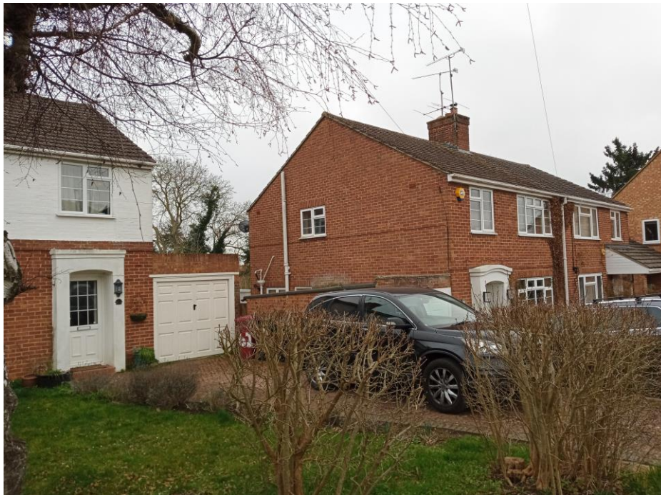
Figure 1: Existing side elevation - viewed from the neighbouring front garden (site visit 21 Feb 2023)
