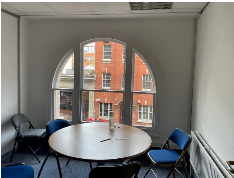
Image 5: internal view of windows on the front facade
