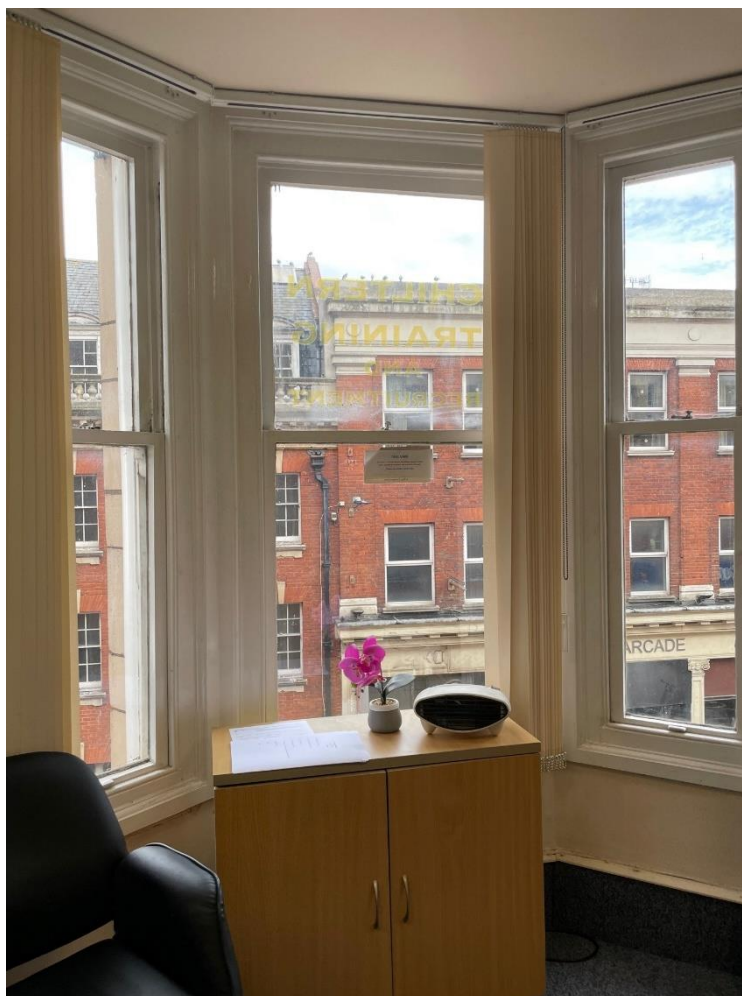
Image 6: internal view of windows on front facade
