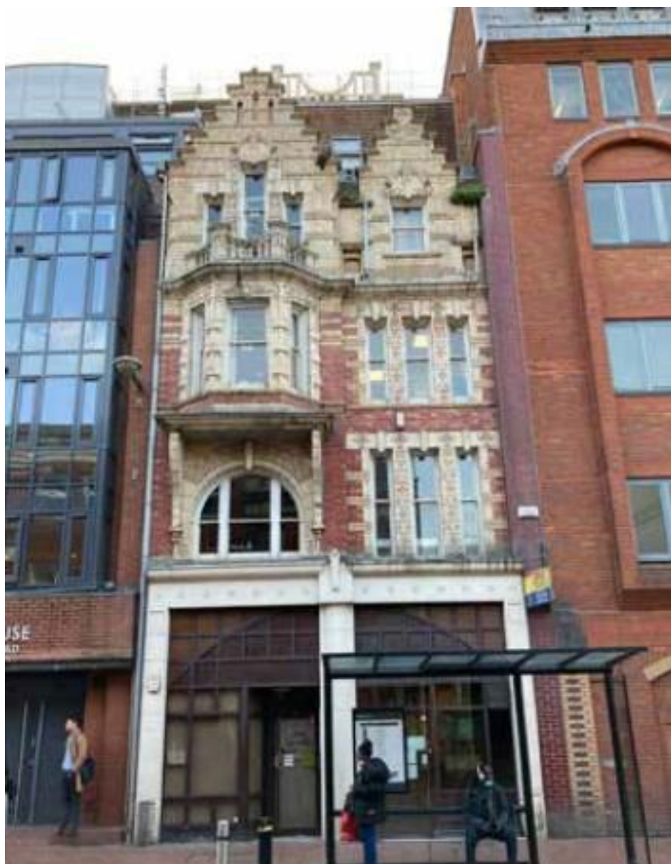
Image 1: Station Road Elevation
