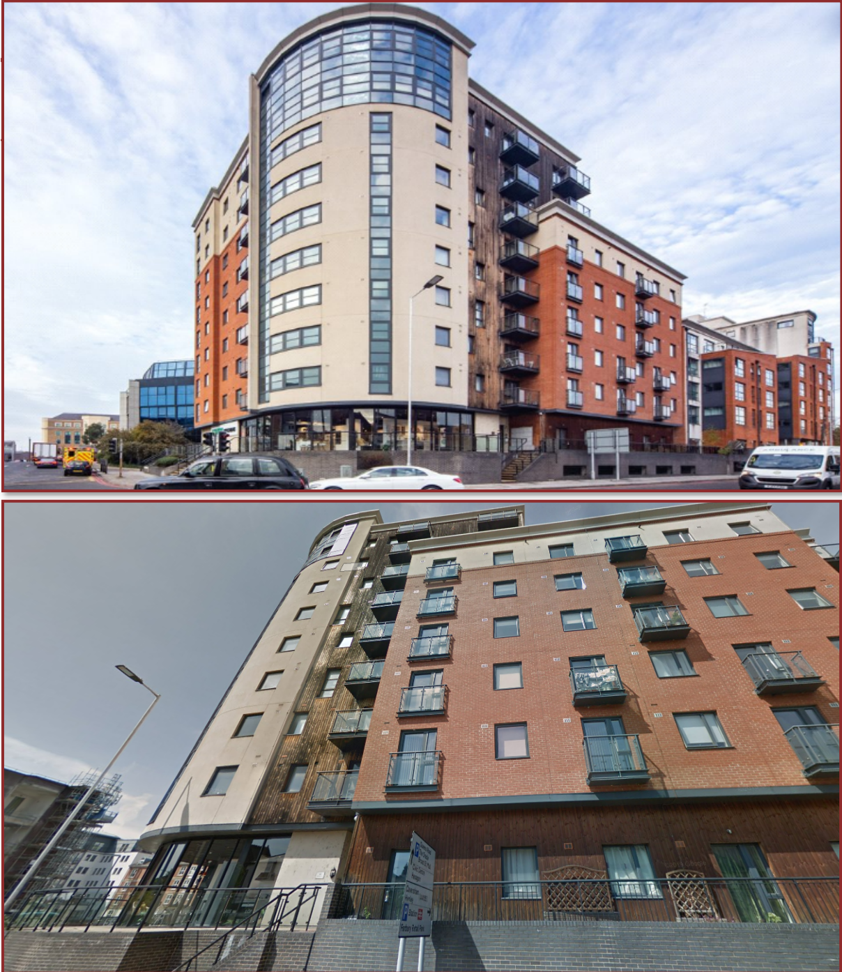
Fig 3. South facing elevation showing masonry brickwork to be remediated
