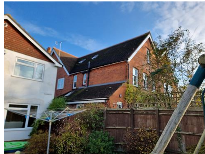
Existing Southern Boundary
