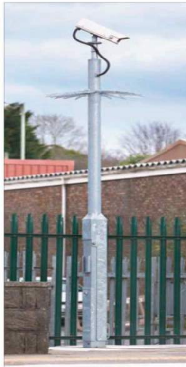
Figure 15 – Altron AW4460/3 4.5m tilt-down SISS /Telecoms pole with anti-climb protection
