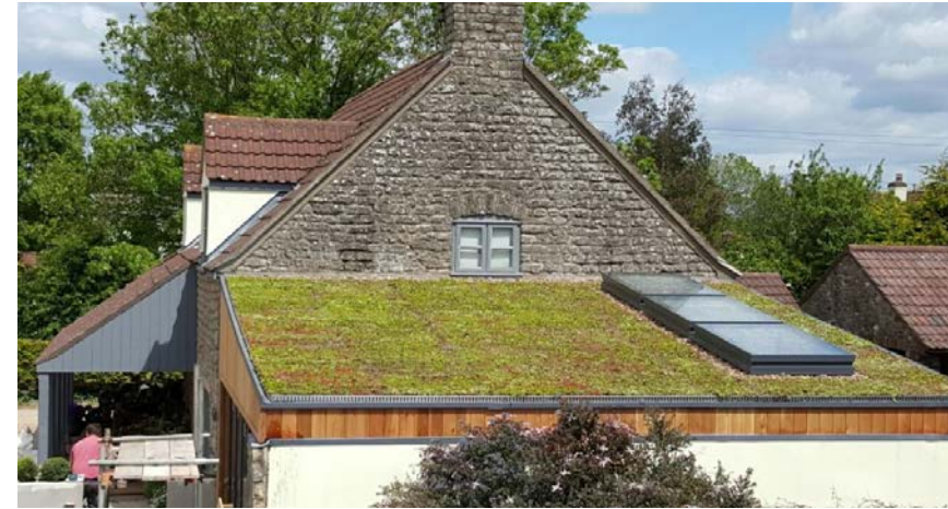
SEDUM ON FLAT ROOF
