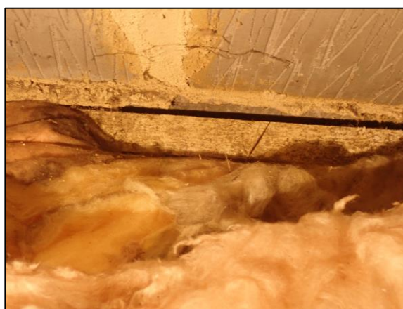
Photo 16 Floor beneath gable end apex
