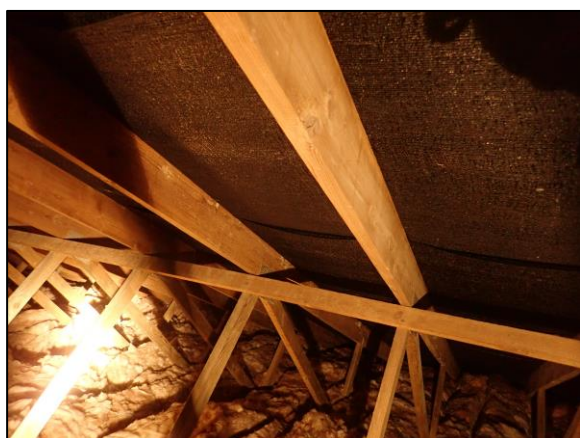
Photo 17 Roofing felt in good condition
