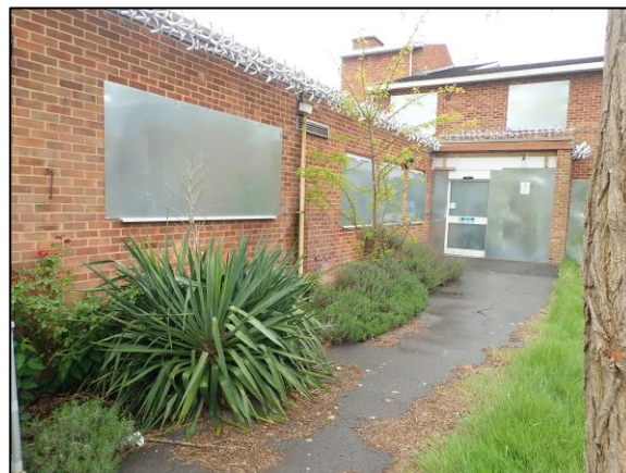
Photo 2 Main entrance area
