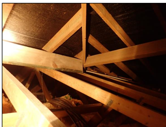
Photo 18 Timber joints and felt in good condition
