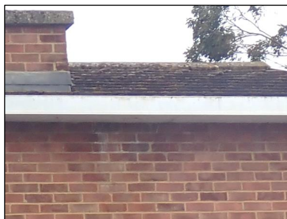
Photo 22 Roof tiles and soffits
