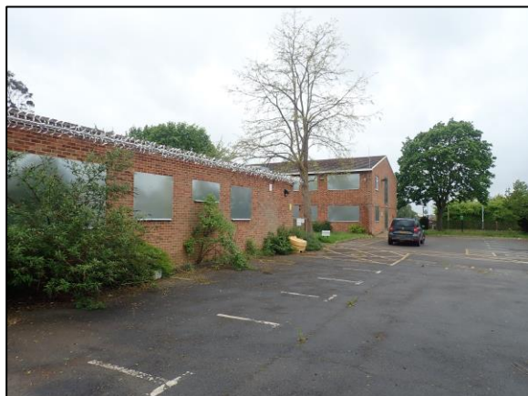
Photo 1 Front of building
