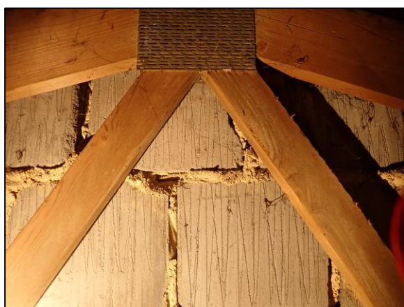
Photo 15 Internal gable wall apex
