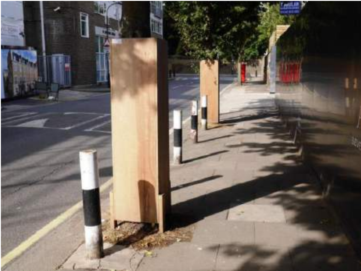
Photo 8: Example of stem box protection.
