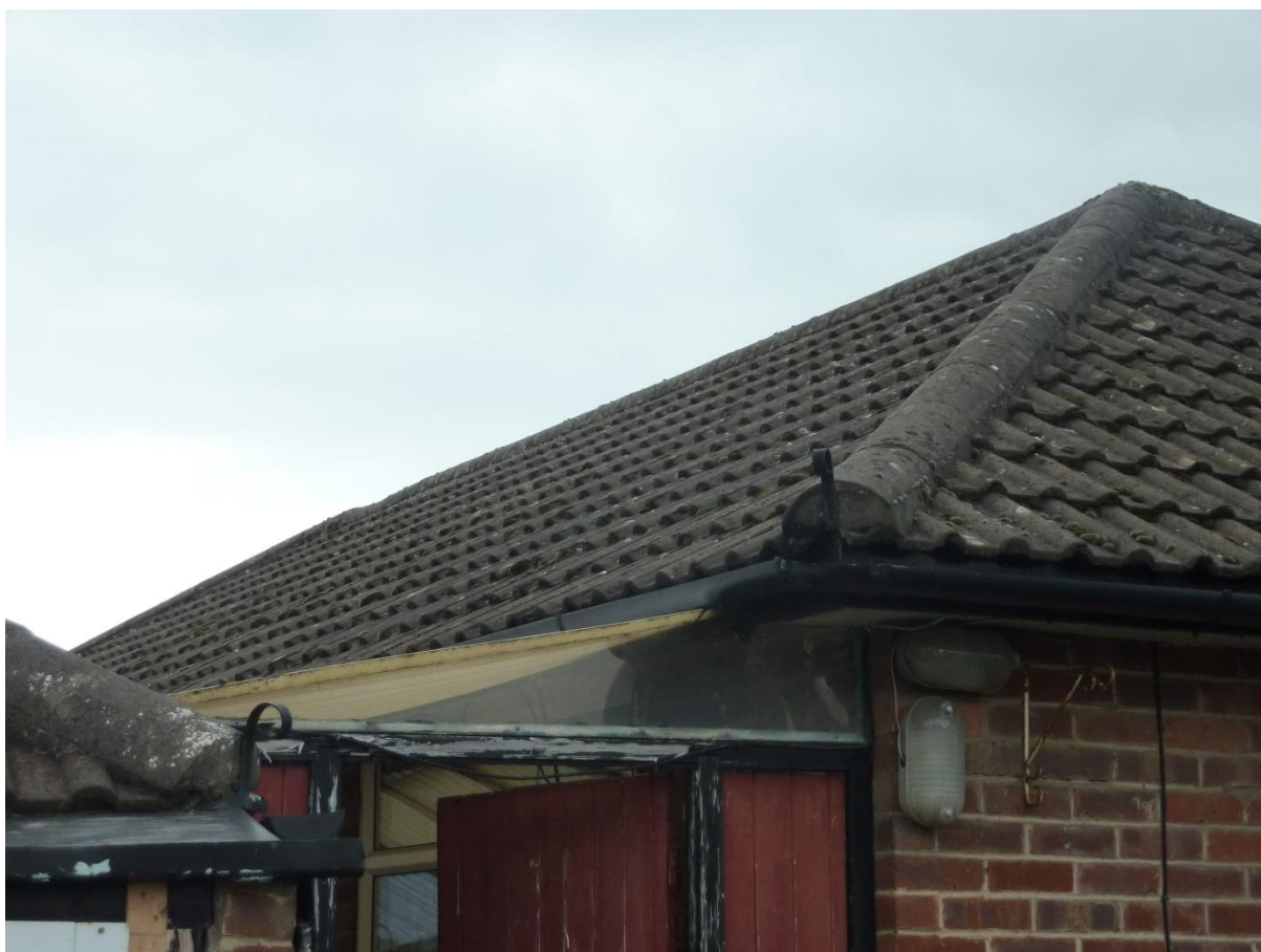
Picture 4: Showing the southern elevation
