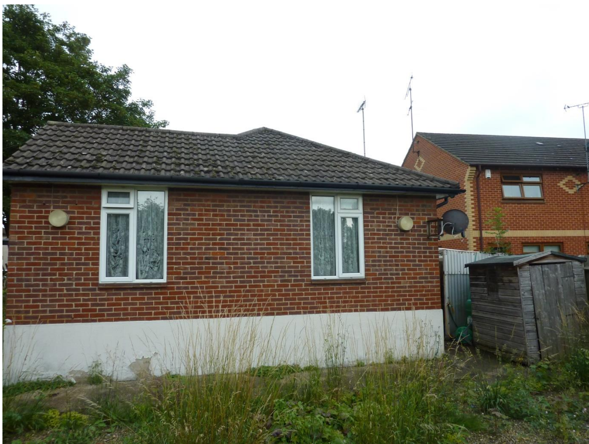
Picture 3: Showing the western elevation
