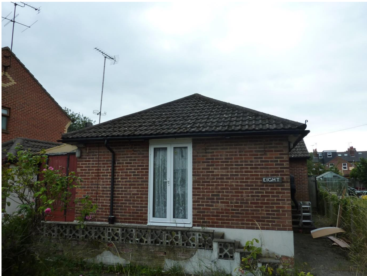
Picture 1: The eastern elevation
