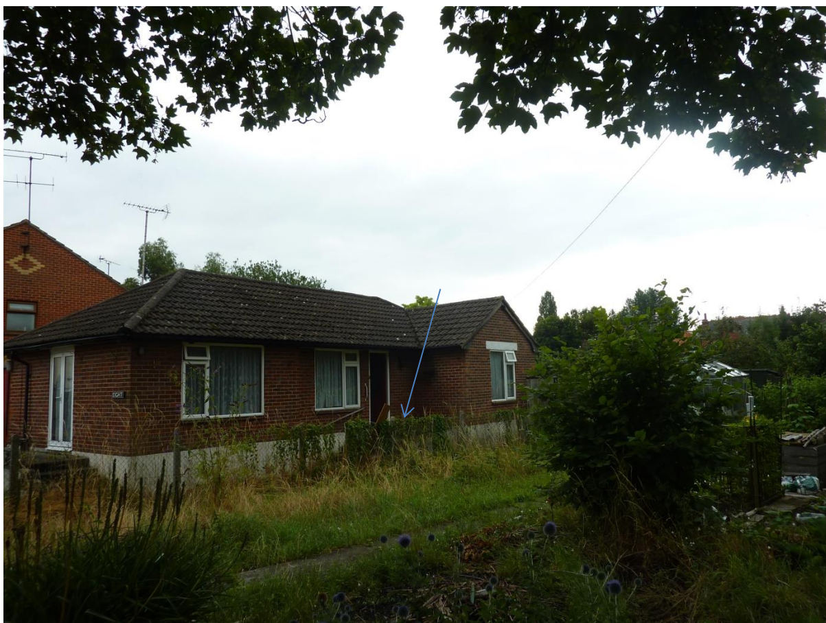
Picture 2: The northern elevation of the building, this picture is taken from the neighbouring plot the chain link fence is the boundary for this property (arrowed).
