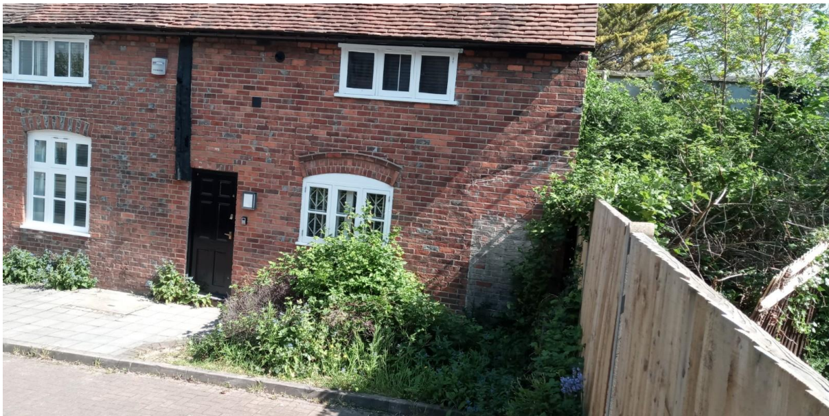
The photo above shows the rear of the LB at 26-28 Southampton Street (looking East)
