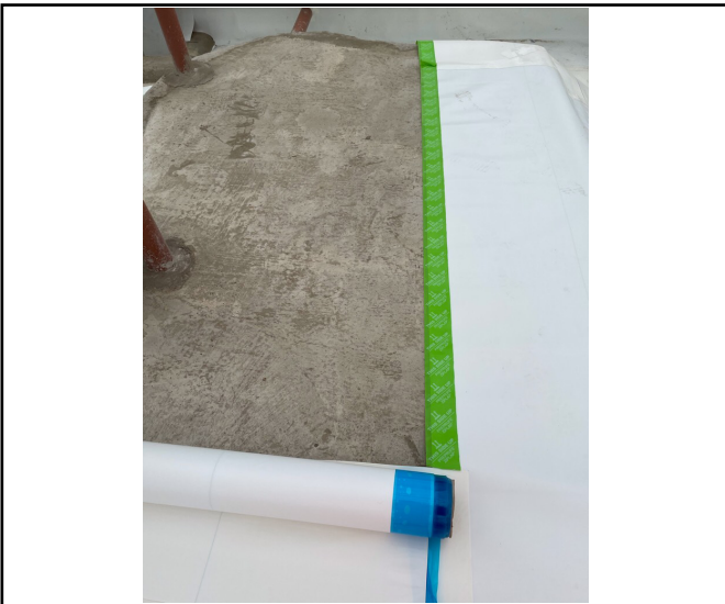
PrePrufe 300R Plus LT membrane preformed taped lap correct way up.
