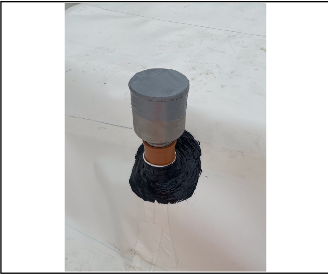
Additional sealed pipe penetration.
