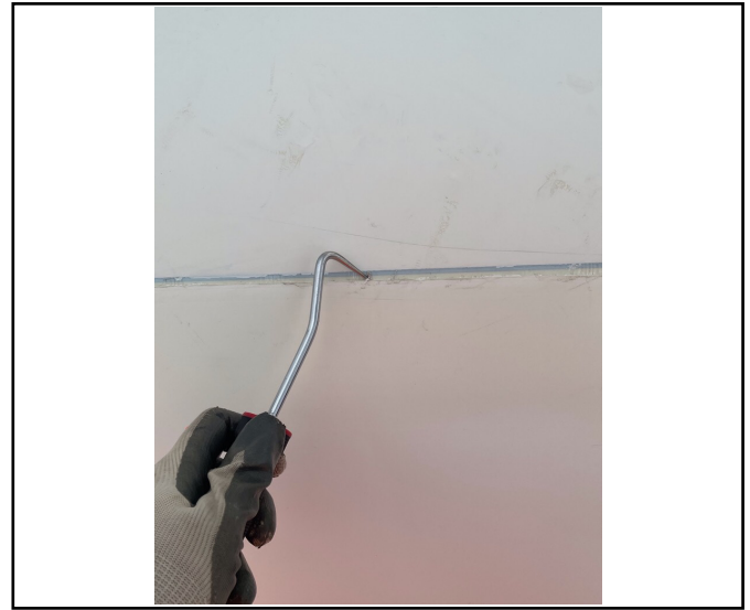
Additional pick and probe test carried out to sealed lap.
