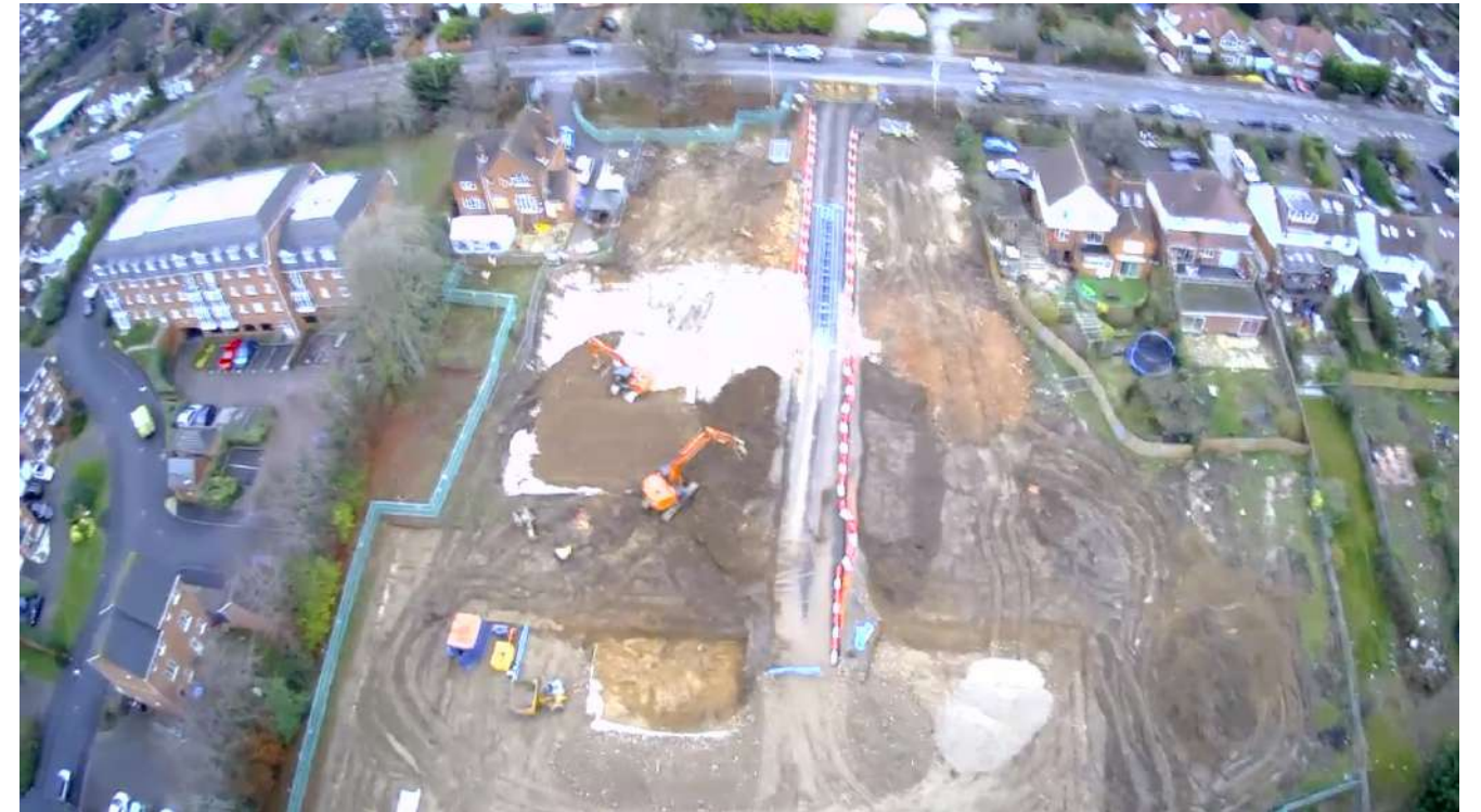
Aerial Image 3: Recent photo showing adjacent scheme under construction.
