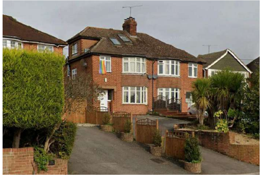
4. The image above is another typical 1930s house with a recent dormer side extension and wrap around roof. This house is constructed of completely red brick.
