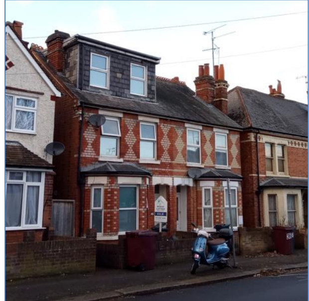
Fig 3. Site photo taken by Case Officer on 27/01/2022.
