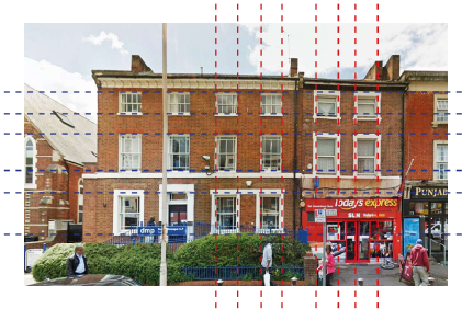
Proportions of residential terraces - 105 Oxford Rd
