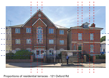
Proportions of residential terraces - 121 Oxford Rd
