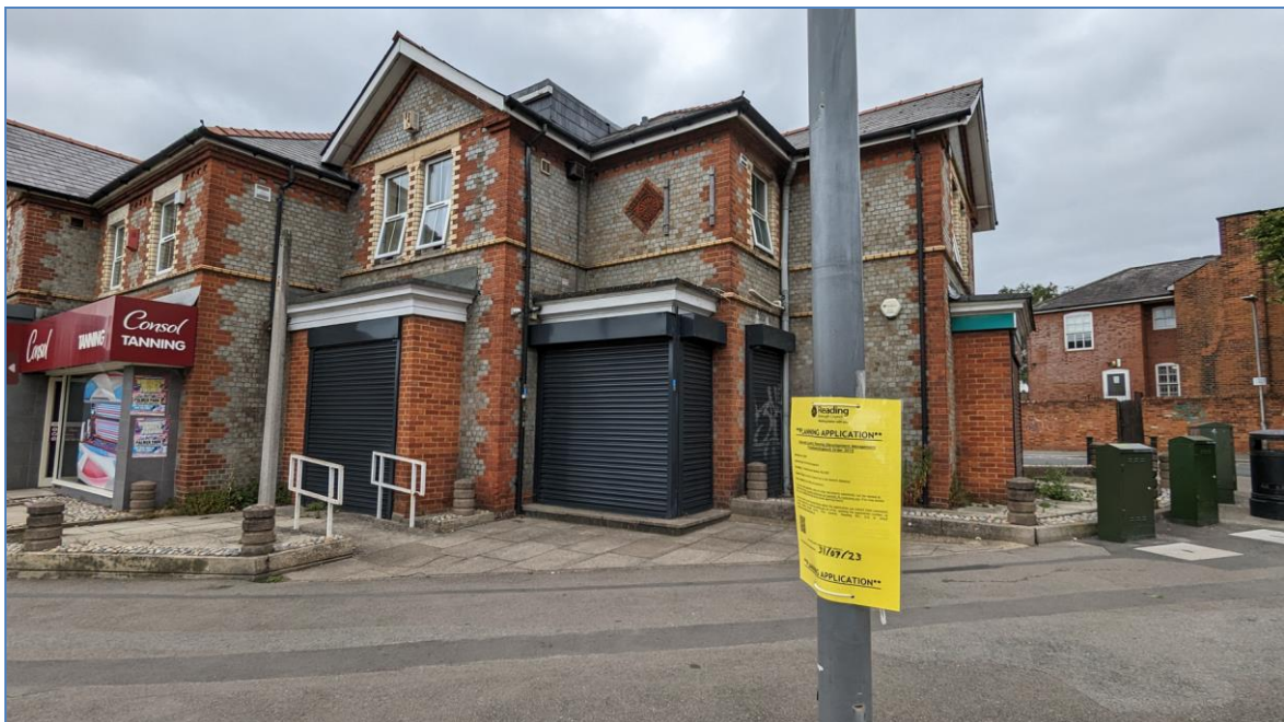
Fig 1. 81 Whitley Street. Site photo taken by Case Officer on 10/07/2023
