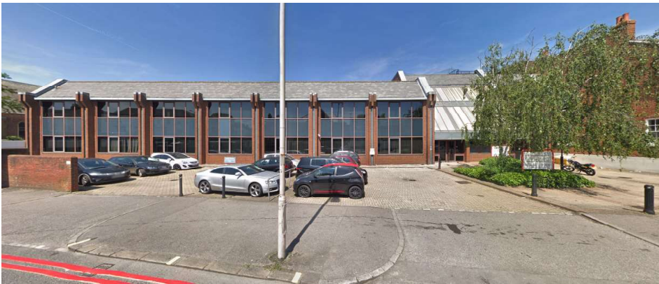
Existing Building - frontage onto Oxford Road
