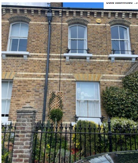
Figure 1: Drainpipe as installed (photo received 11 April)
