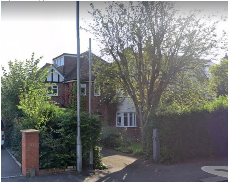
Figure 1: Application Site - Front View
