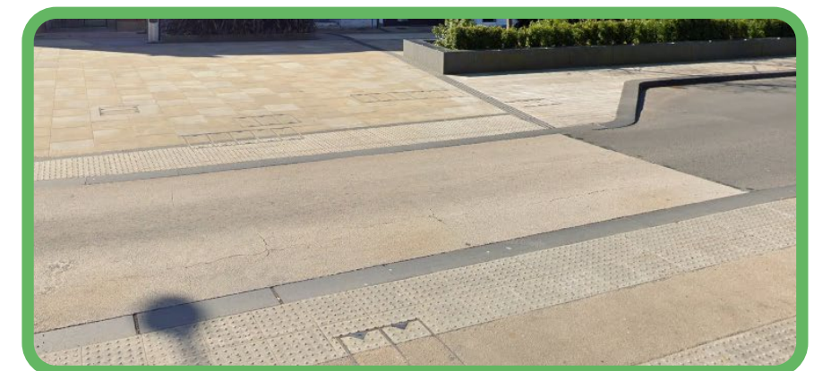
Illustrative examples of pedestrian priority crossing detailing.- Raised Crossing (Copenhagen Crossing), Tactile roadway surfaces, Surfacing change and build-out at crossing.
