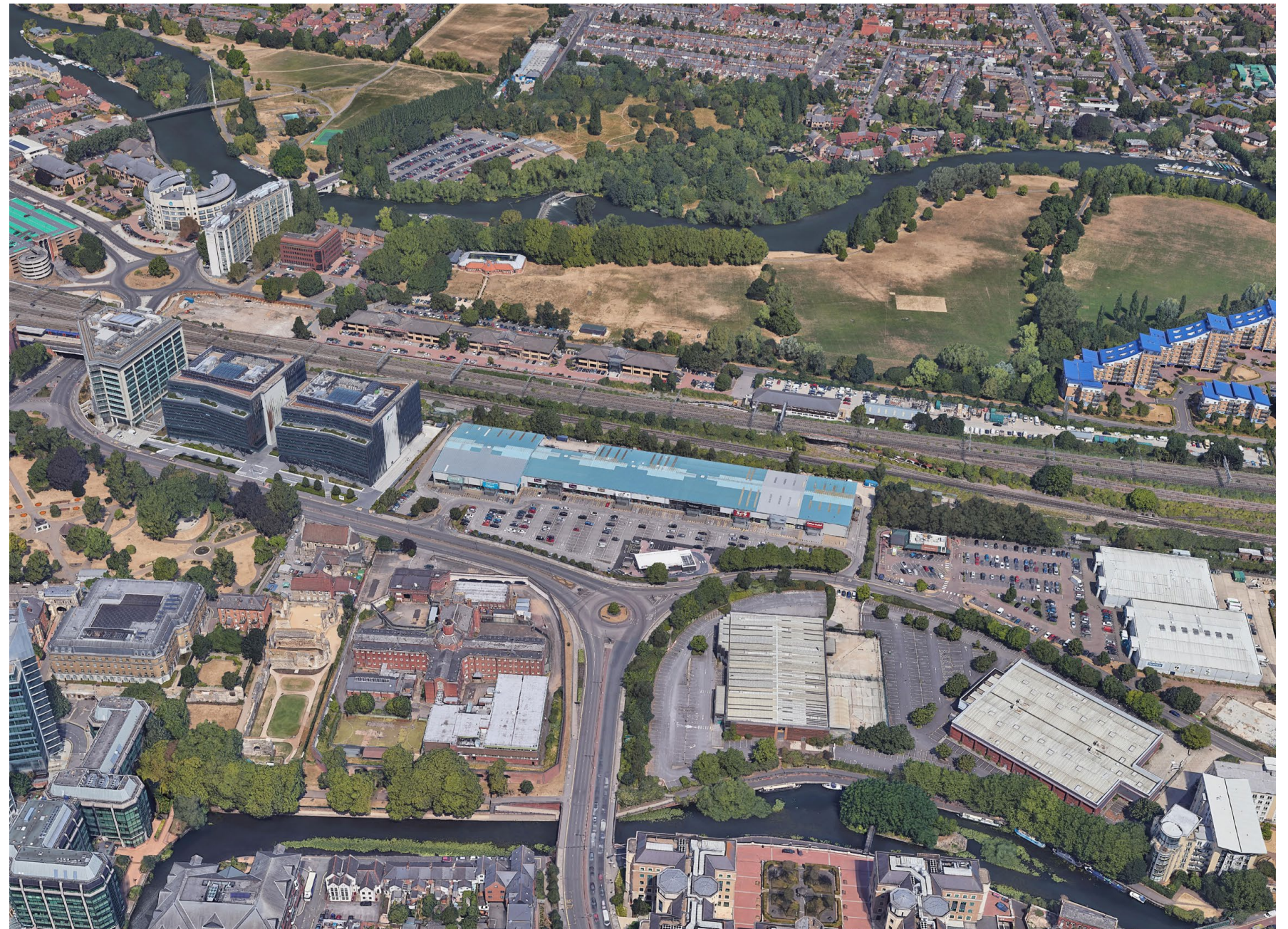
Existing Aerial View
