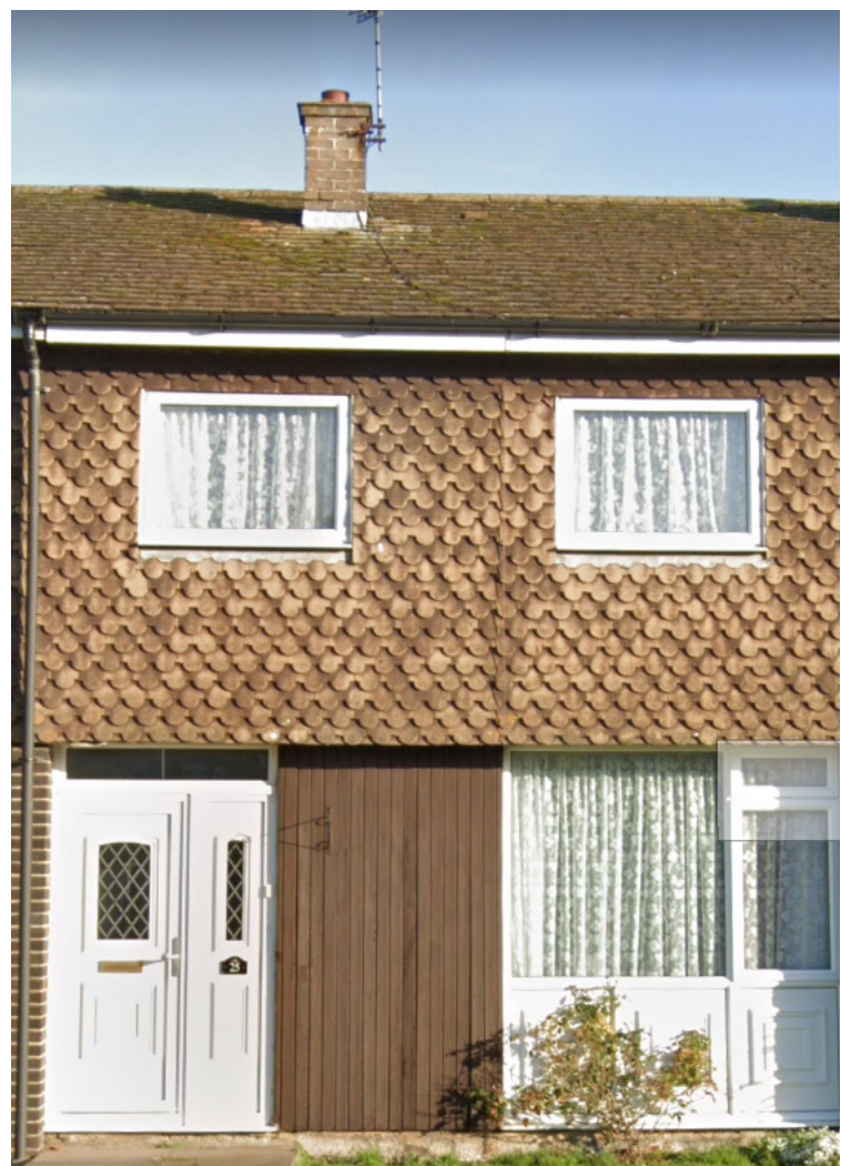
Scalloped tiles - Hexham Road, Reading (Google Maps)
