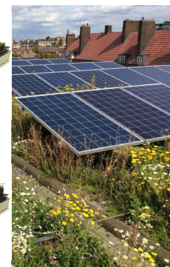
Typical rooftop combining PV & biodiverse planting
