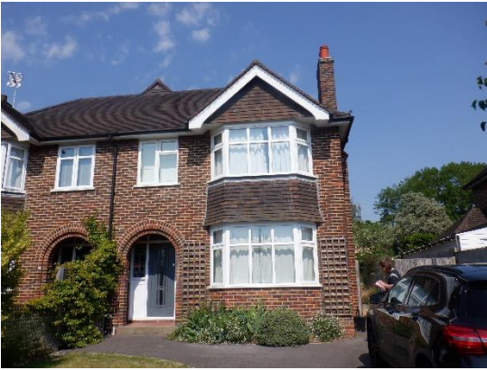
1. Front of property viewed from west.
