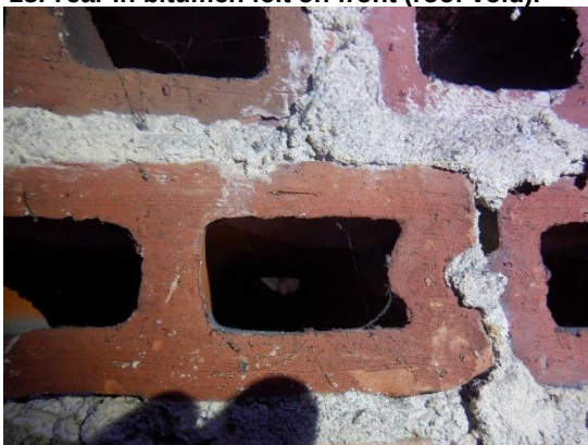
15. Hollow bricks in party wall (roof void).
