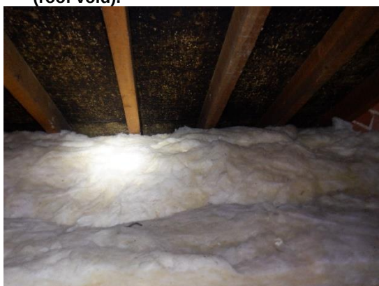
11. Fibreglass insulation filling eaves (roof void).
