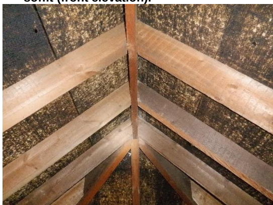
9. Hessian-reinforced bitumen roofing felt (roof void).
