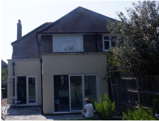
2. Rear of property viewed from east.
