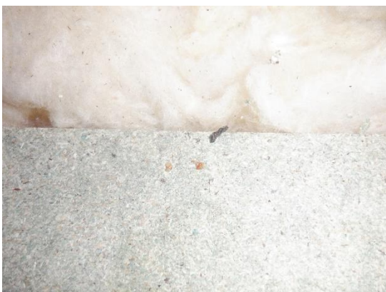
17. Medium-sized bat dropping on floor (roof void).
