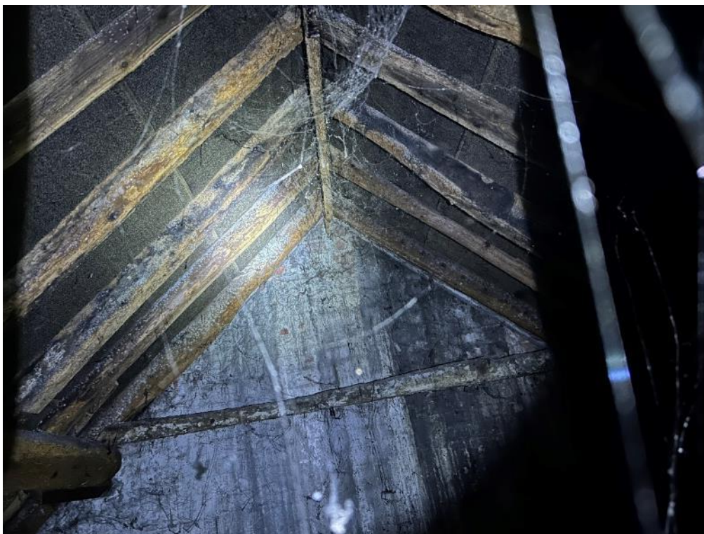
Photograph 44: Barn, entirety of tiles lined with felt
