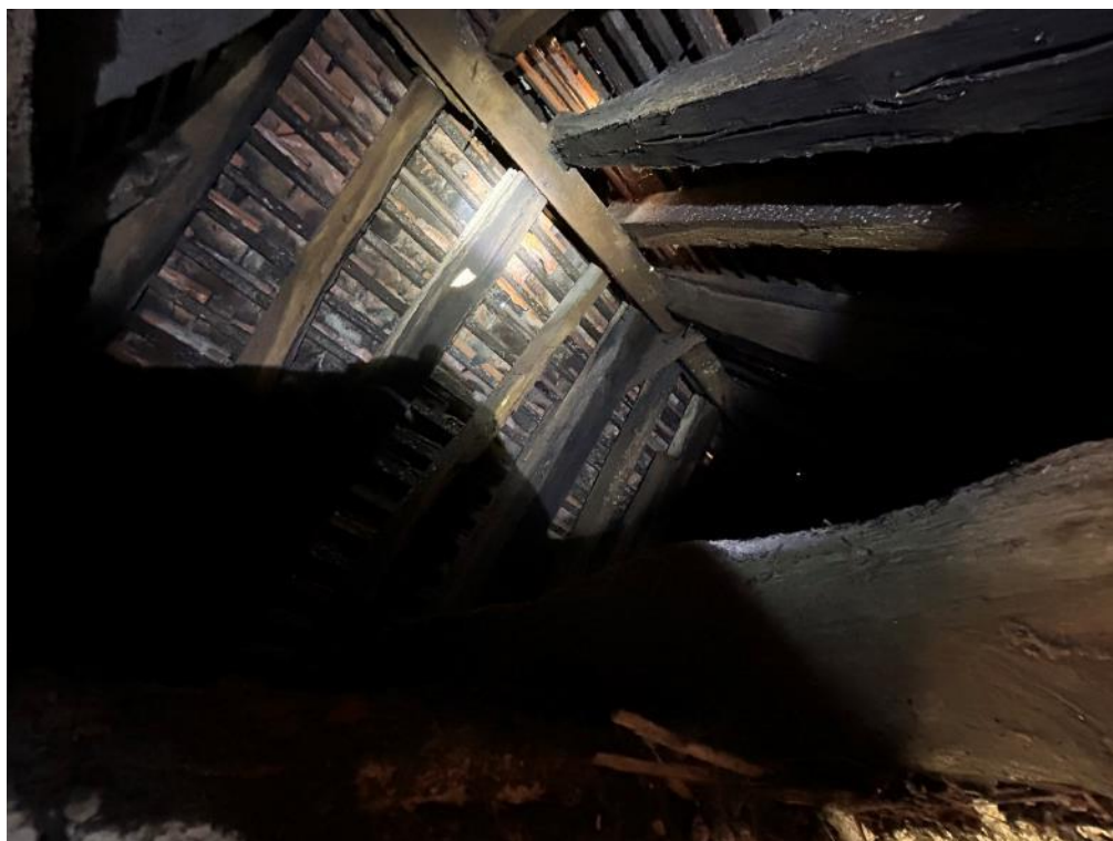
Photograph 15: Main Pub, sealed void above loft space room 1
