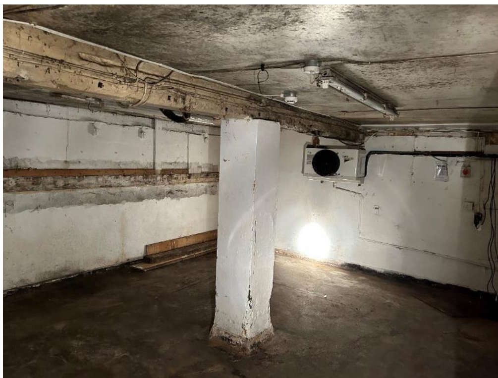
Photograph 18: Main Pub, cellar beneath original structure
