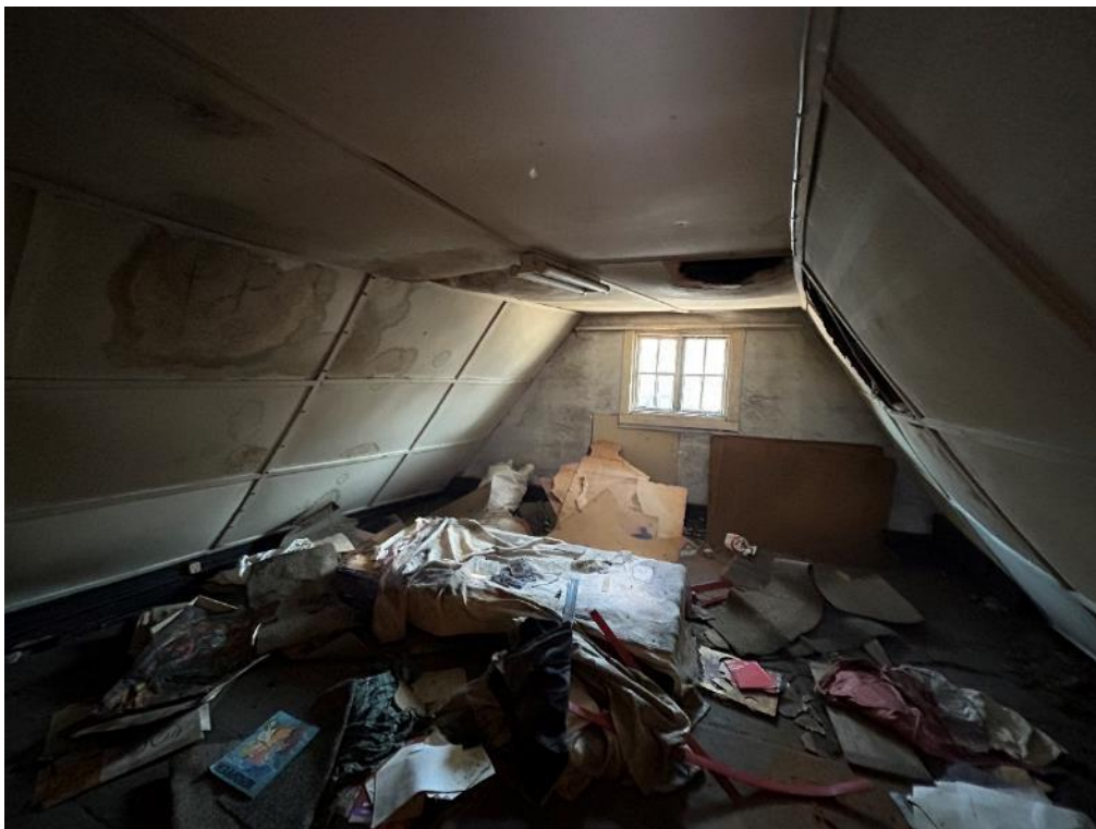
Photograph 13: Main Pub, loft space room 2
