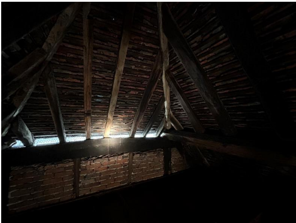
Photograph 11: Main Pub, loft space (L2)
