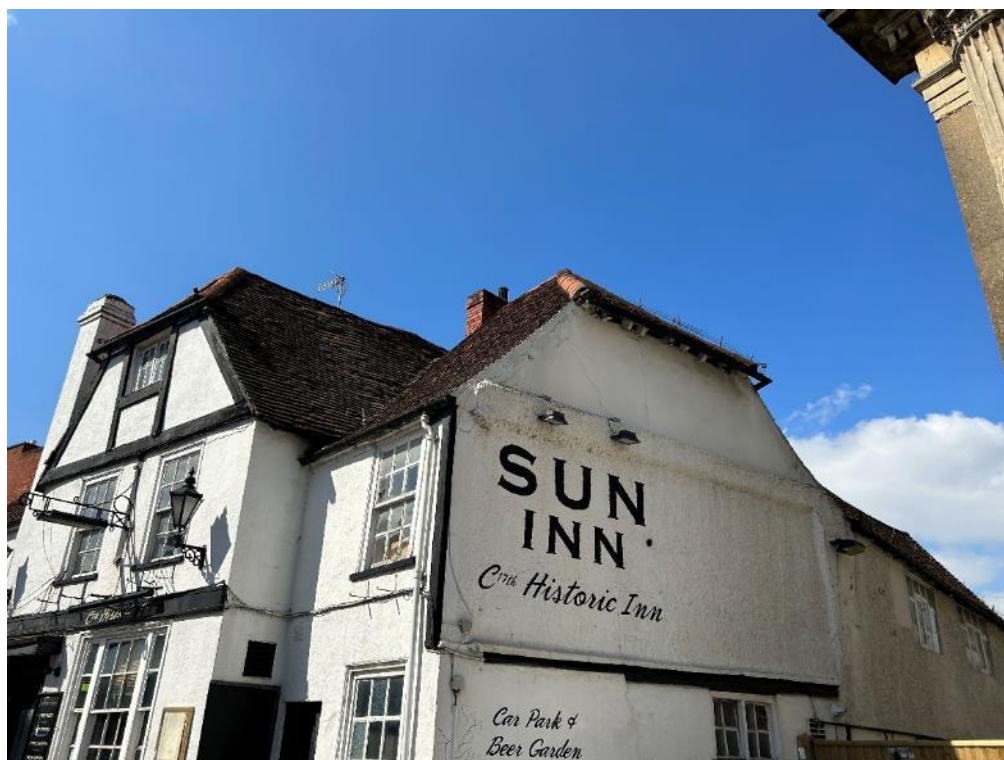
Photograph 4: Main Pub, southern and eastern elevations
