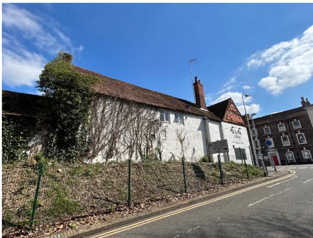
Photograph 6: Main Pub, western elevations
