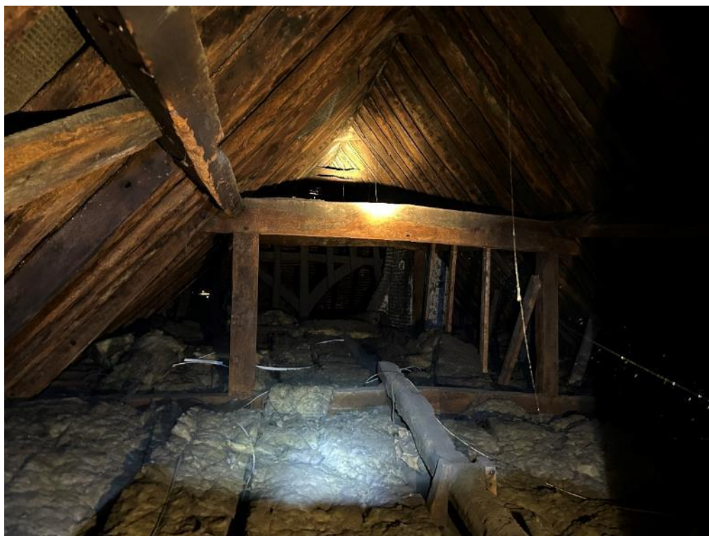
Photograph 9: Main Pub, loft space (L1) – Viewed from centre of roof, facing chimney stack (looking south)
