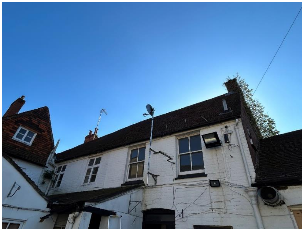
Photograph 8: Main Pub, eastern elevations 'court yard' facing
