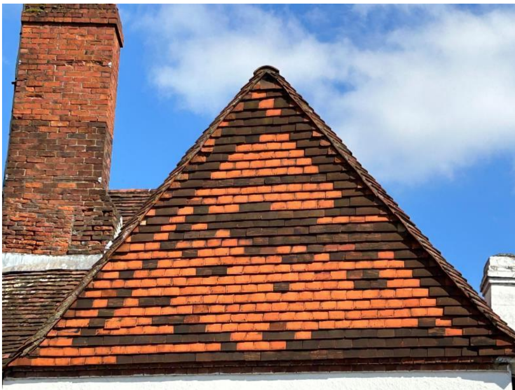
Photograph 32: Main Pub, hanging tiles, western elevation
