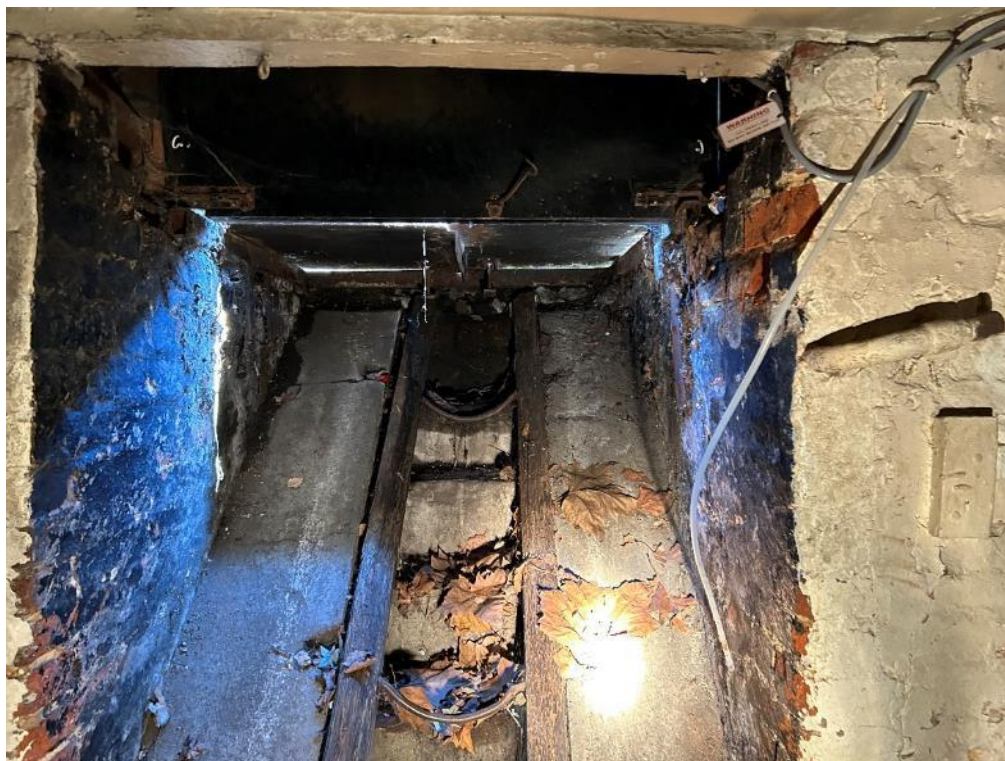
Photograph 20: Main Pub, hatch from cellar onto Castle Street
