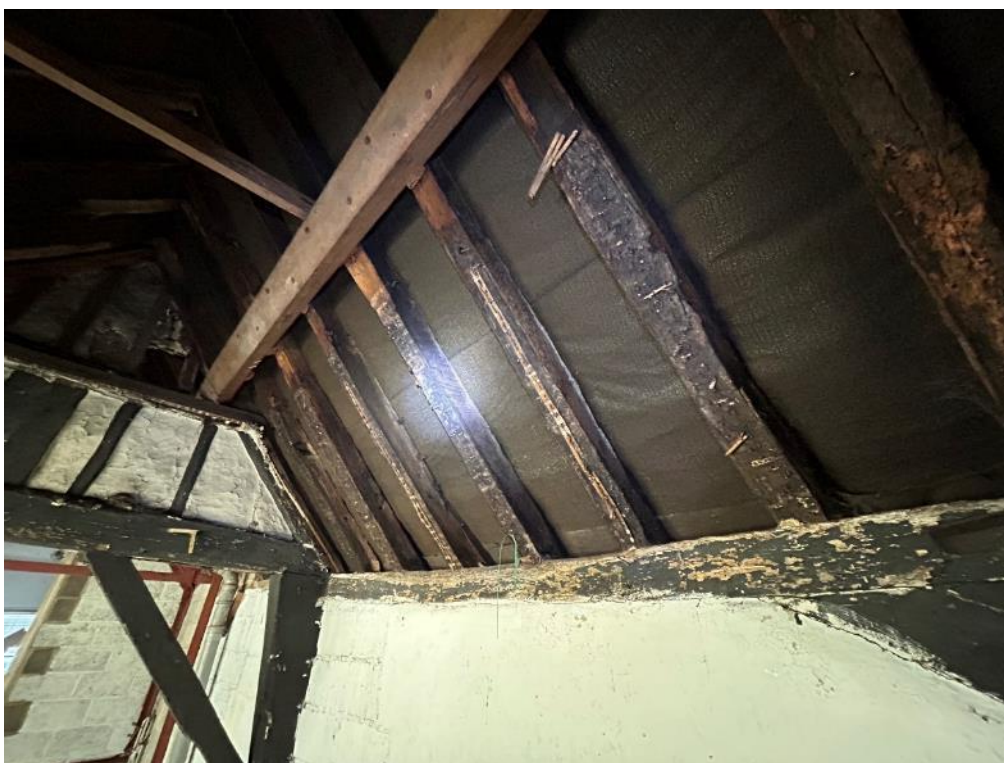
Photograph 39: Main Pub, internal of room 3, tiles were felt lined
