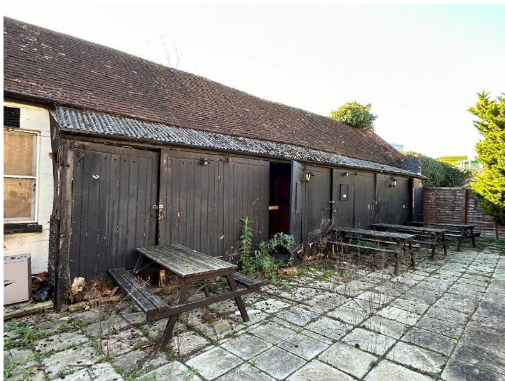
Photograph 22: Barn, eastern elevation with wooden lean-to
