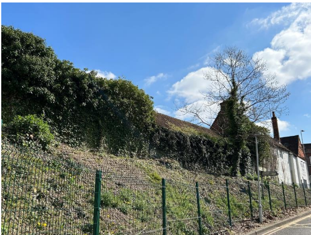
Photograph 45: Main Pub, Barn, adjacent wall, ivy lattice
