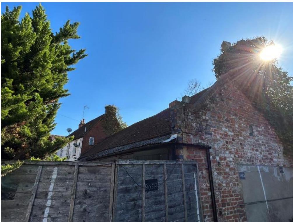
Photograph 21: Barn, northern and eastern elevations
