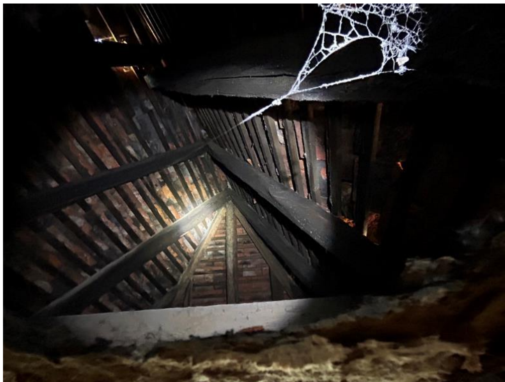
Photograph 16: Main Pub, sealed void above loft space room 2
