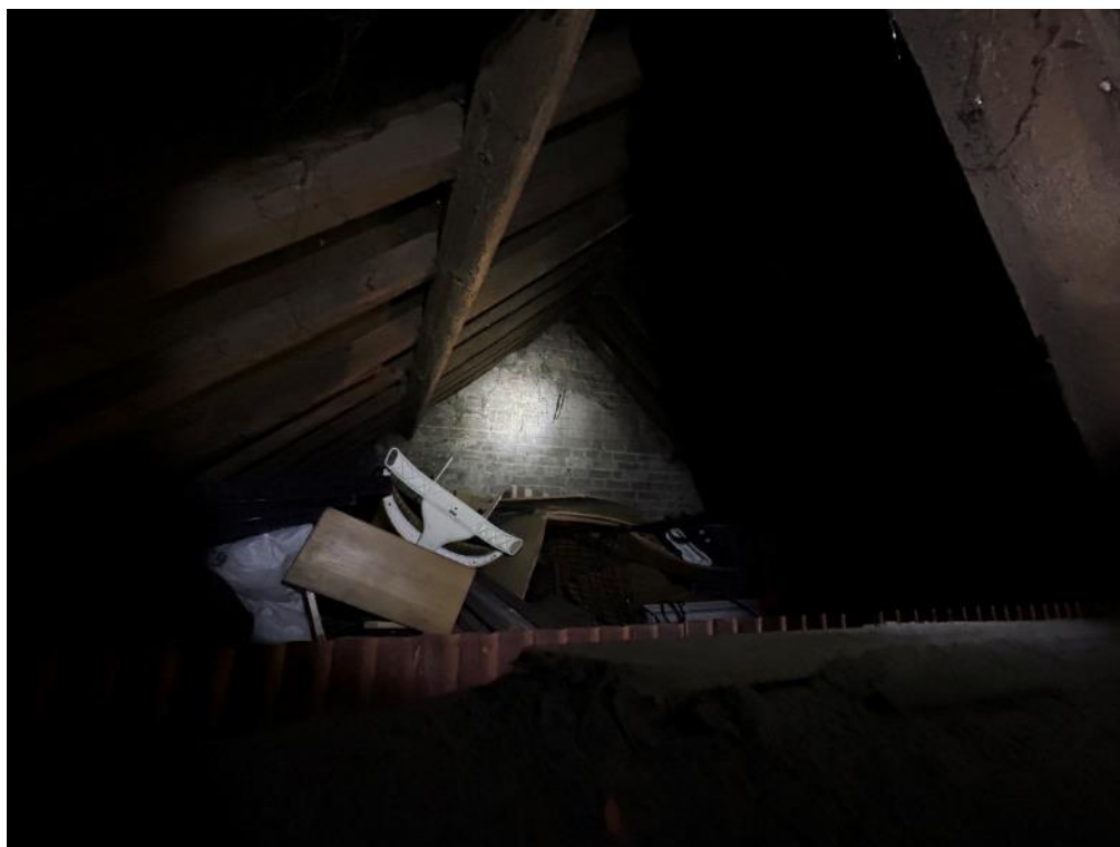
Photograph 26: Barn loft space, northern extent viewing from south
