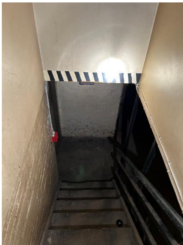
Photograph 19: Main Pub, internal staircase leading to cellar
