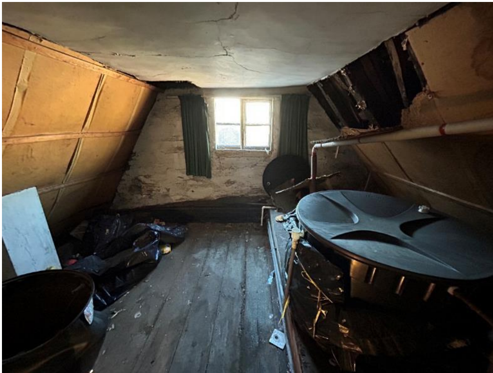
Photograph 12: Main Pub, loft space room 1
