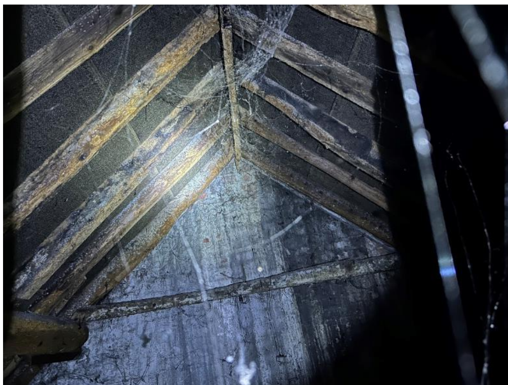
Photograph 29: Barn loft space, southern extent viewing from south
