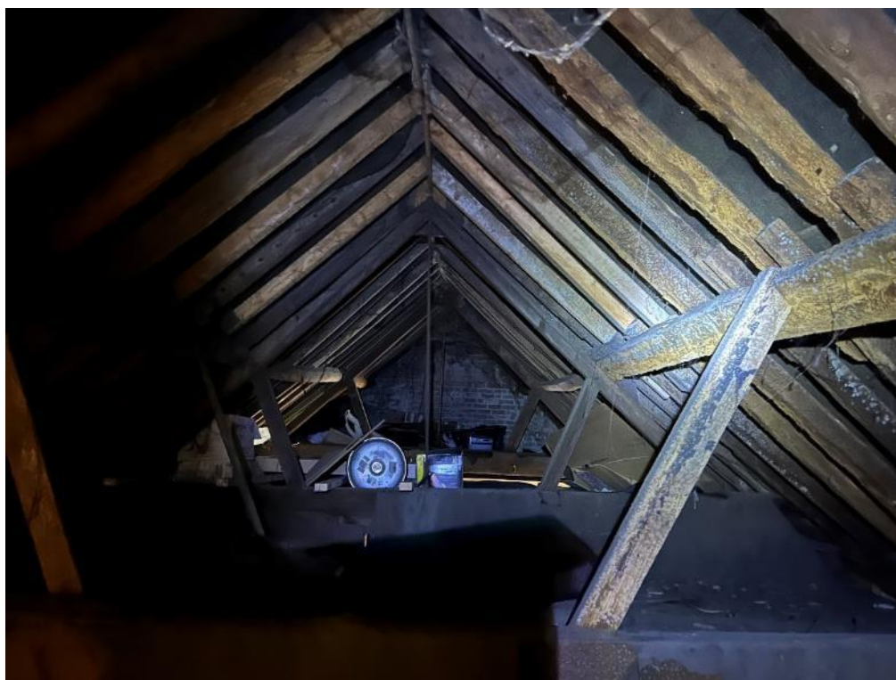
Photograph 27: Barn loft space, central area viewing from south looking north
