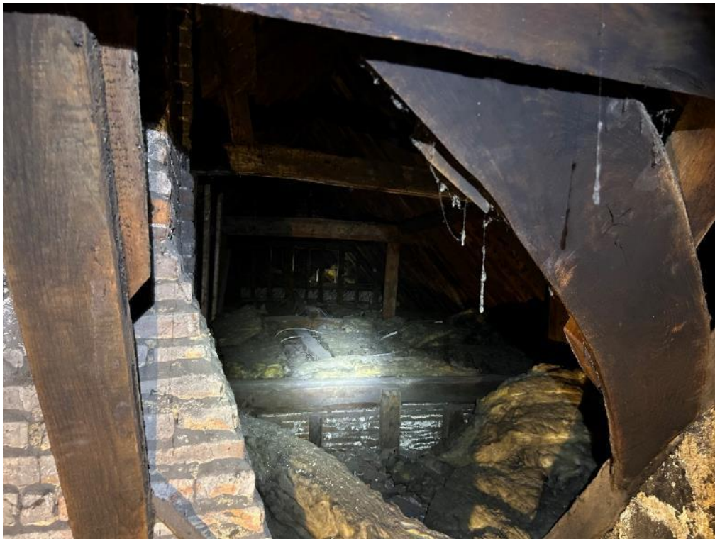
Photograph 10: Main Pub, loft space (L1) – Viewed from chimney stack, facing north
