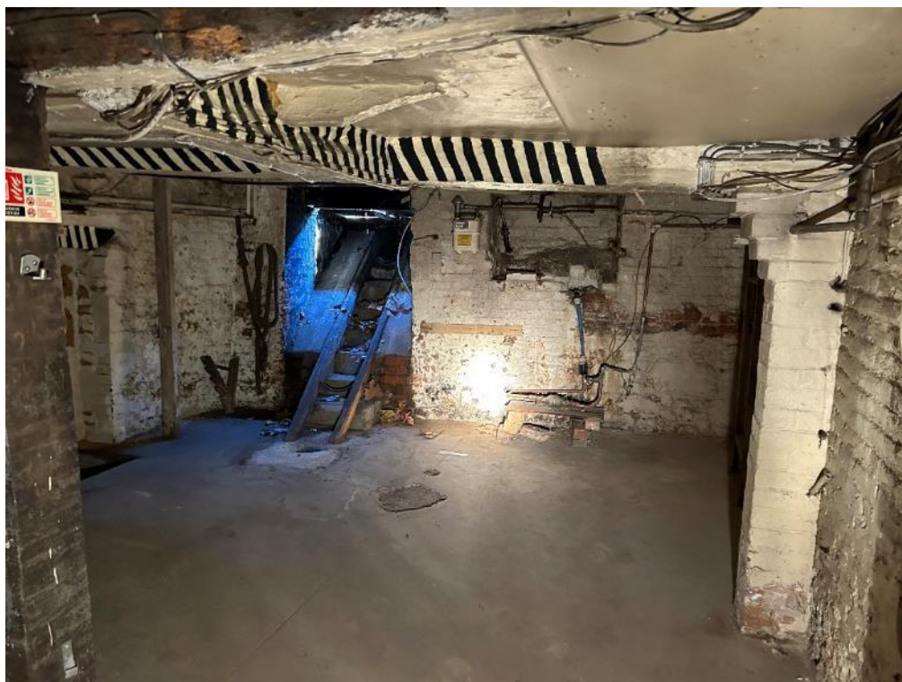
Photograph 17: Main Pub, cellar beneath original structure
