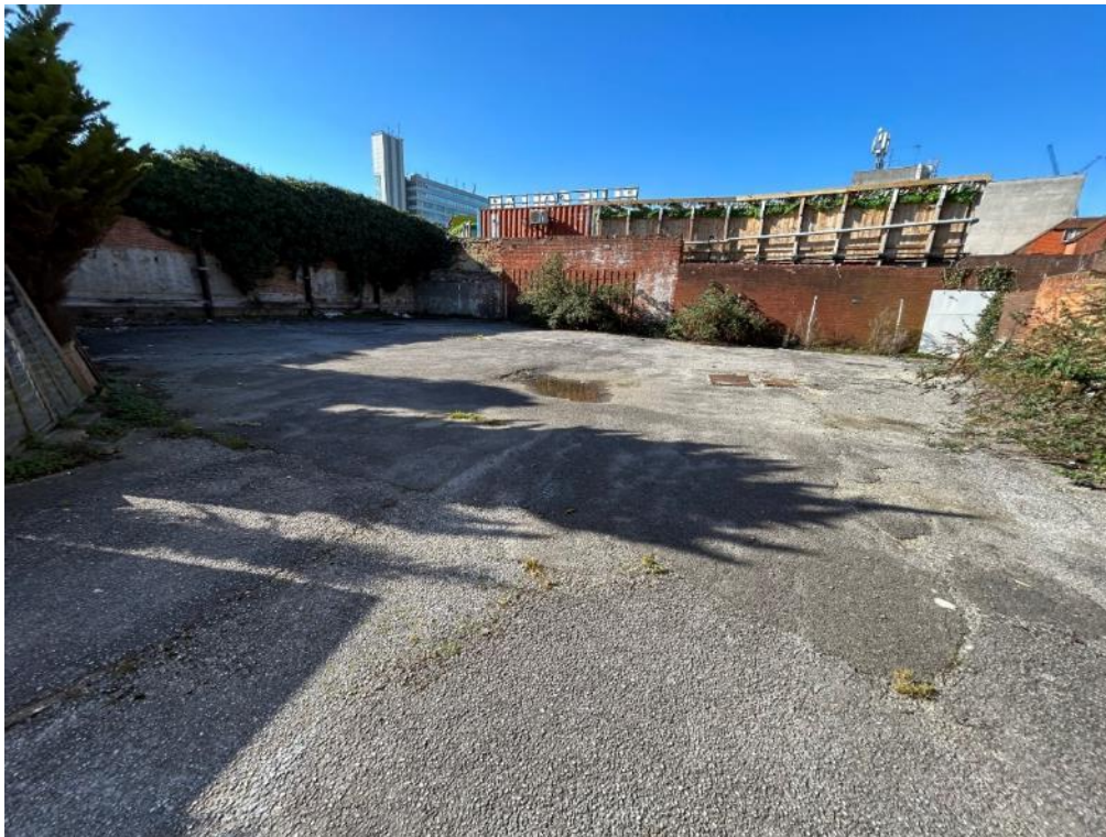
Photograph 1: Large tarmac car park
