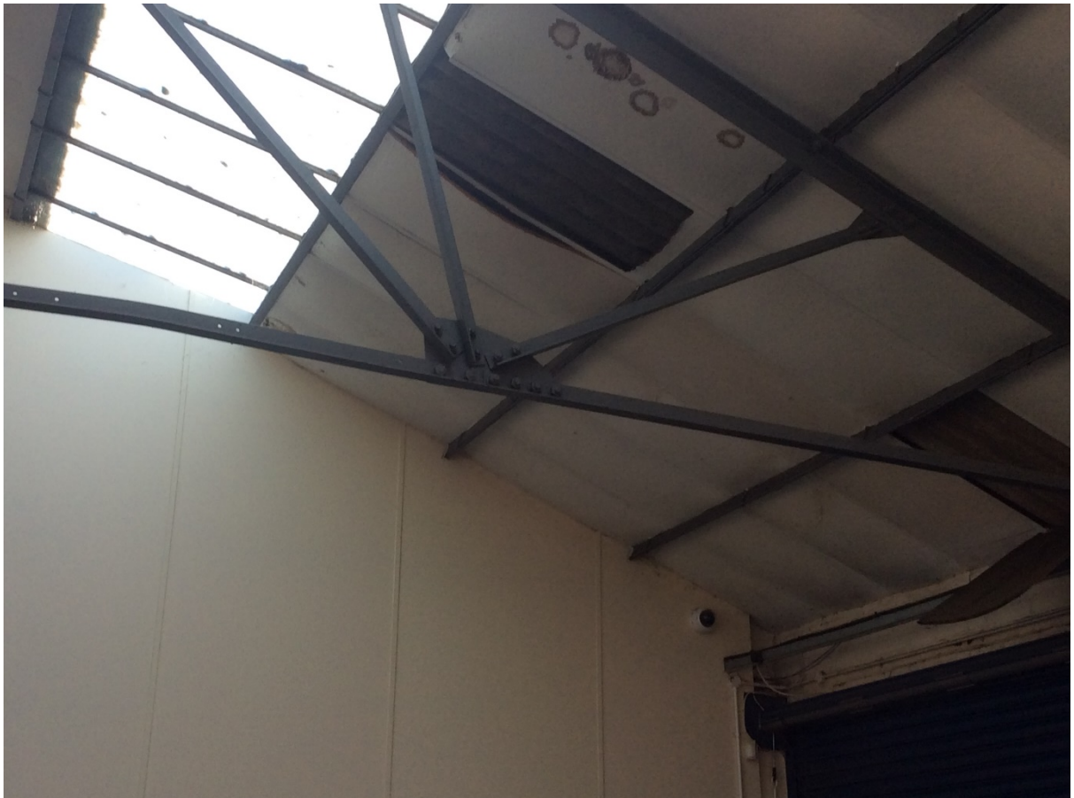
Figure 3. Interior of workshop looking east.
