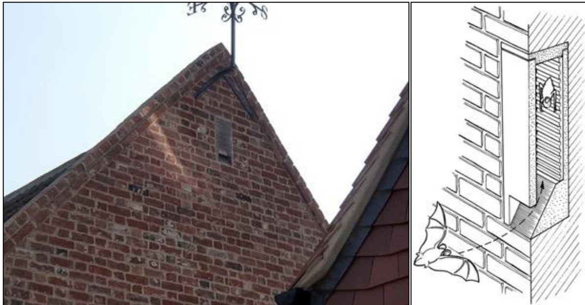
Figure 5. Left – A bat tube integrated into a brick wall. Right – a cross section diagram of a bat tube.
