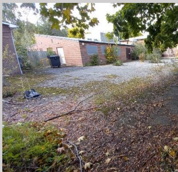
Photograph 15: Southern aspect of Building 3 slight pitched roof
