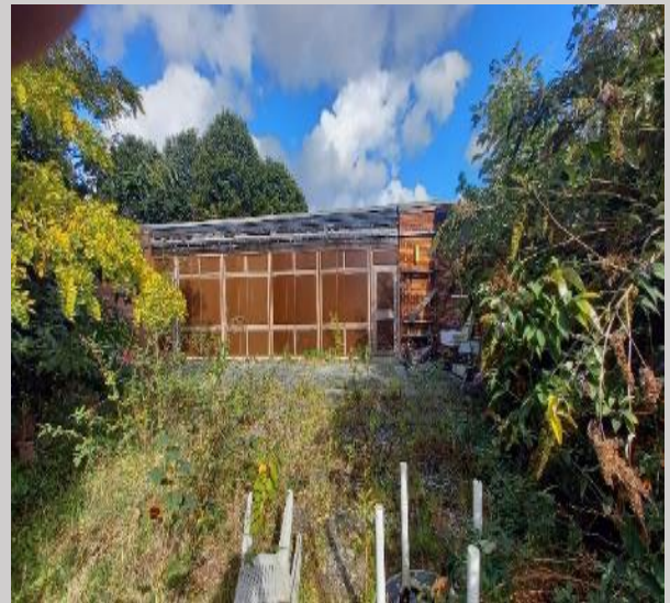
Photograph 22: Exterior windows of Building 3 covered by metal grates
