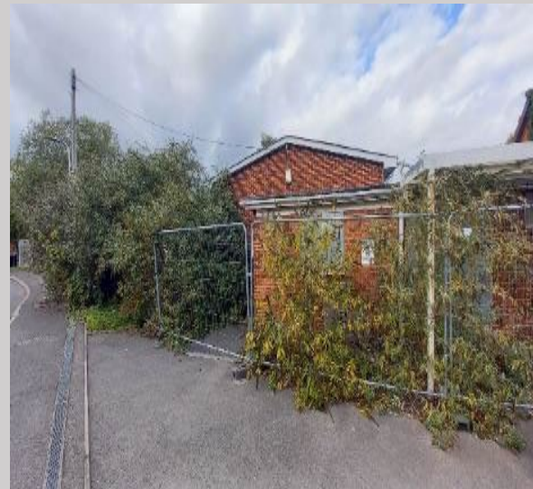
Photograph 14: Southern aspect of Building 2
