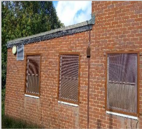
Photograph 21: Southern aspect of Building 3 with wood soffit
