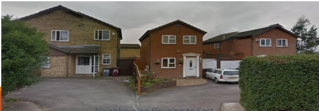
Neighbouring Housing to East
