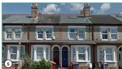
5 Paired first floor windows
