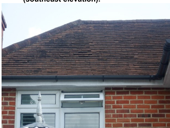
5. Ridge and hip tiles securely mortared (rear elevation).
