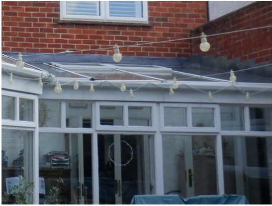
13. Lead flashing along conservatory (rear elevation).
