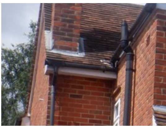
6. Tight lead flashing around chimney at southeast gable (front elevation).
