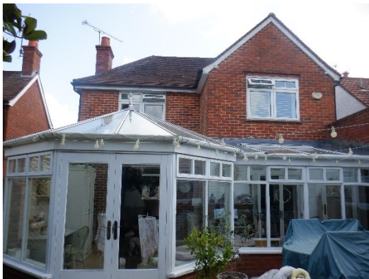
2. Rear of house viewed from southwest.
