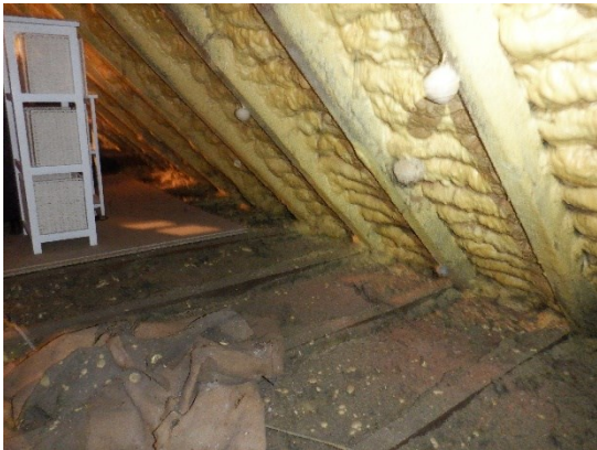
17. Fibreglass floor insulation (roof space).
