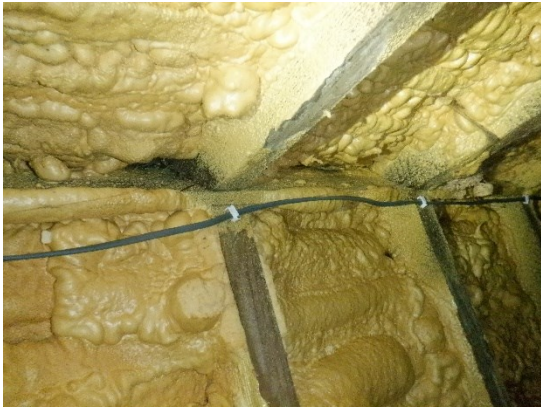
19. Ridge beam covered in spray foam insulation (roof space).
