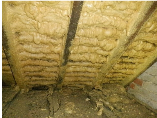
16. Roof lined with spray foam insulation (roof space).
