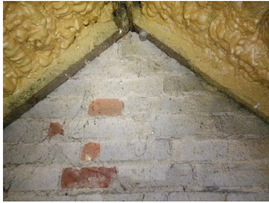
20. Spray foam sealed against gable wall (roof space).
