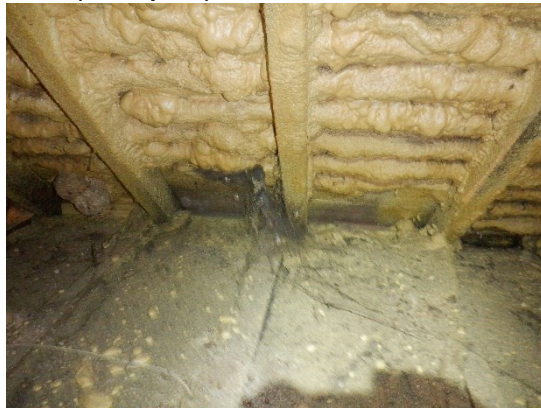
18. Timber associated with chimneys visible in eaves (roof space).
