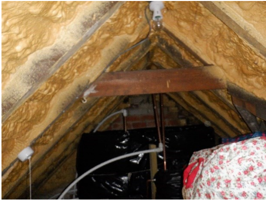
15. Covered water tank (roof space).
