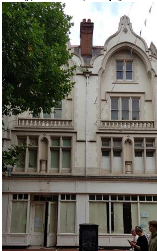
Figure 1: Existing front elevation (photo by agent 2/9/22)
