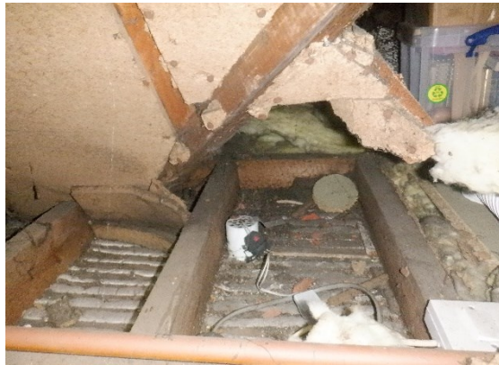
20. Part boarded floor over fibreglass insulation.
