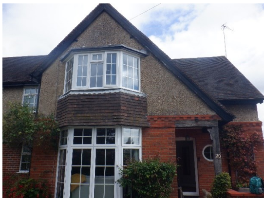
1. Front of property viewed from the southwest.
