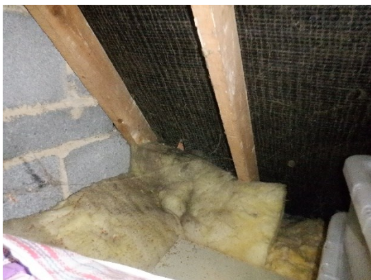
25. Part boarded over fibreglass insulation.
