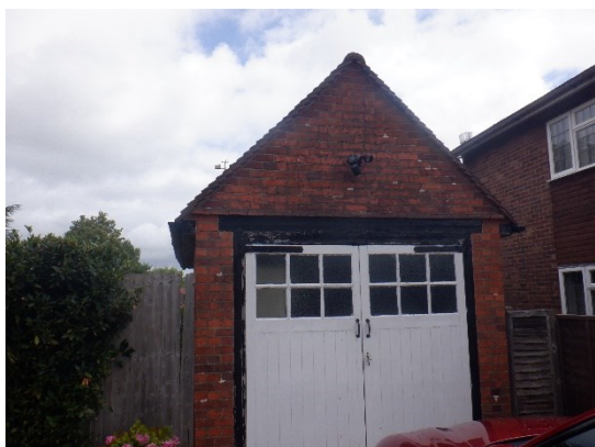
3. Front of the garage viewed from the southwest.
