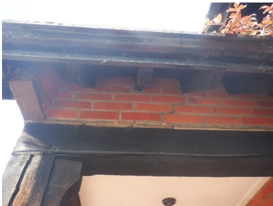
11. Soffit mostly tight to brickwork throughout.
