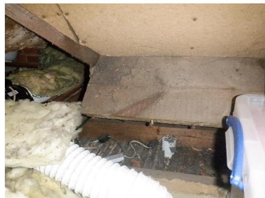
22. Eaves open and part covered with wooden planks.
