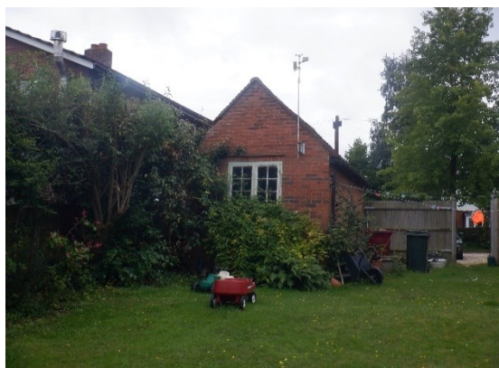
4. Rear of the garage viewed from the northeast.
