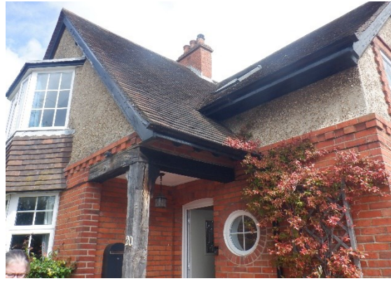
8. Verge mortar of front gable intact.
