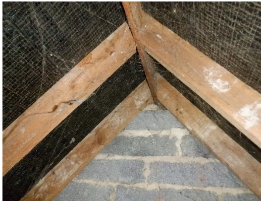
23. Bitumen reinforced felt liner.
