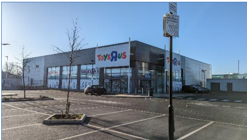
Fig 1. Front of Unit 6, Proctor End South. Photo taken by case officer on 06/02/2023
