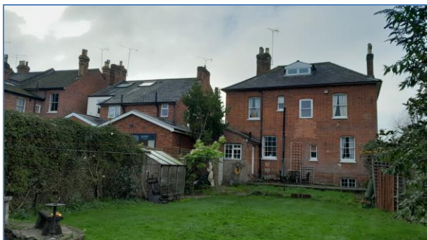
Fig 2. Rear of 85 Hamilton Road. Site photo taken on 30/11/2022.
