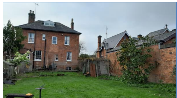
Fig 3. Rear of 85 Hamilton Road. Site photo taken on 30/11/2022.
