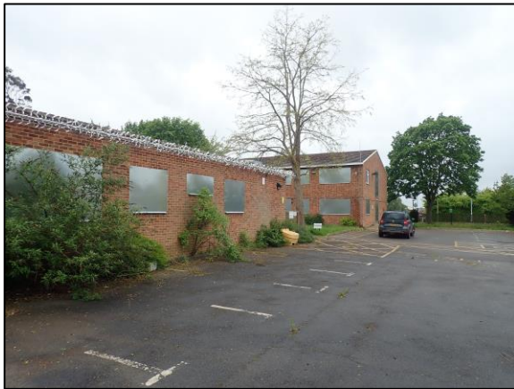
Photo 1 Front of building (prior to demolition)
