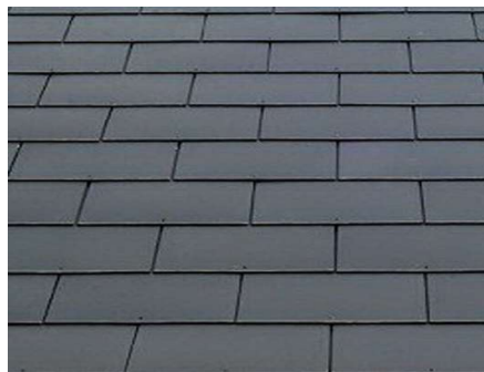
Slate tiles, reclaimed where possible to match existing
