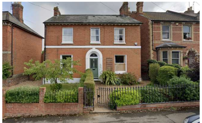
Figure 17. 87 Hamilton Road - Google Maps
