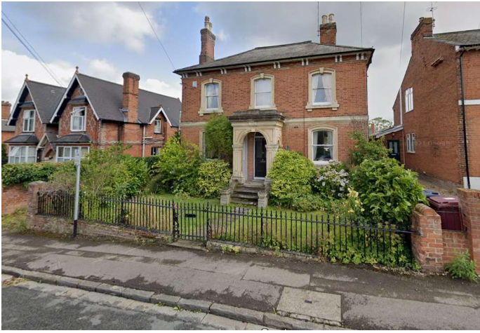
Figure 10. 85 Hamilton Road - Google Maps
