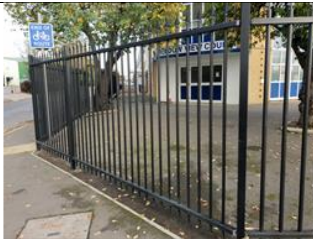
Illus. 18: The railing are slightly wider than the tomb so that it can be seen through, and not over-power the setting. The details are similar but do not copy the original square railings. Round railings have been selected for the new fence.
