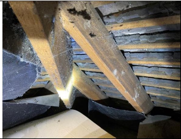
Photo 8 Area beneath PRFs
