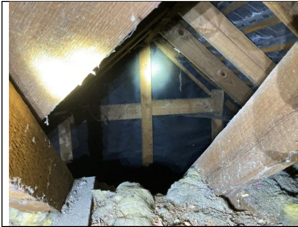
Photo 7 West gable interior
