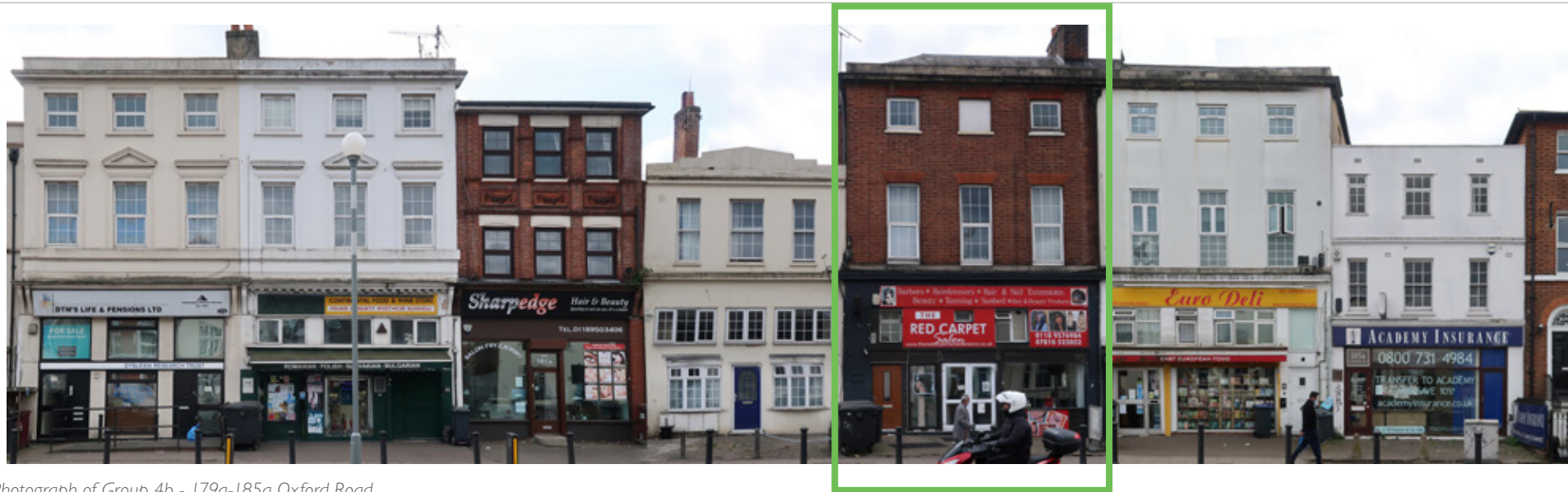
Photograph of Group 4b - 179a-185a Oxford Road. No. 183a has been highlighted
