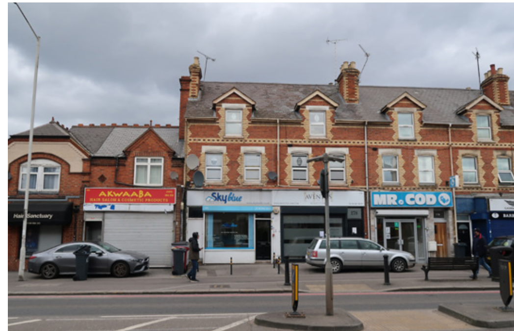
Late Victorian terraced development next to the railway bridge.
