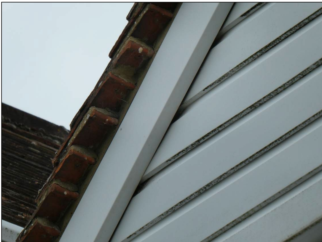
Figure 11. PVC cladding on dormer window. 46 Grosvenor Road, Caversham. 12.09.23
