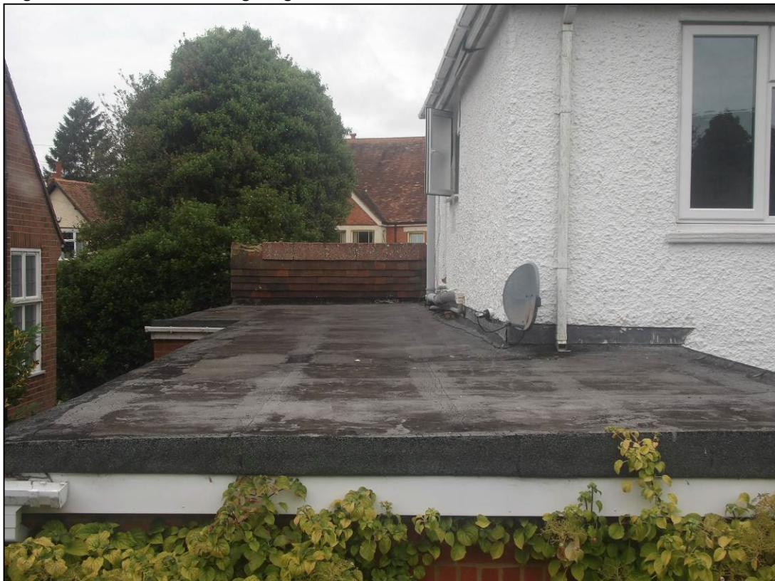
Figure 13. Flat section of garage roof. 46 Grosvenor Road, Caversham. 12.09.23
