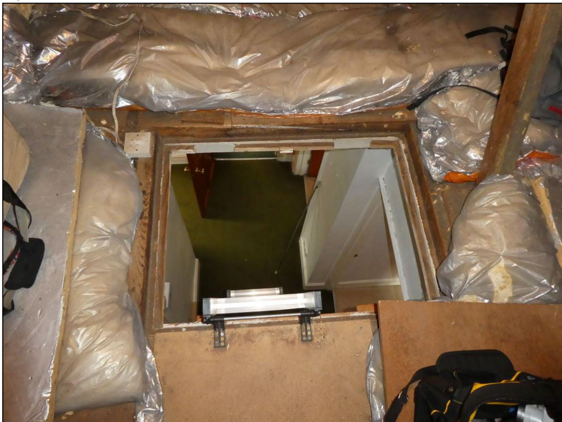
Figure 14. Loft hatch. 46 Grosvenor Road, Caversham. 12.09.23
