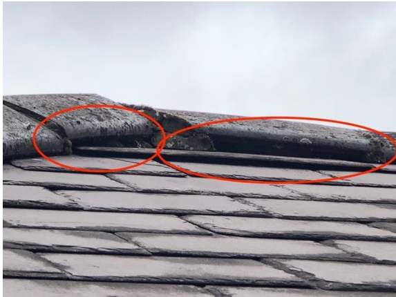
Photo 15: Missing ridge tile pointing and lifted slates.
