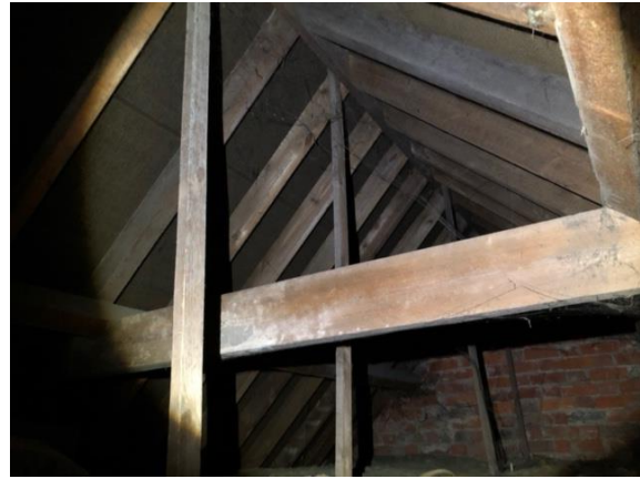
Photo 10: One of the roof spaces – well-sealed with no daylight.
