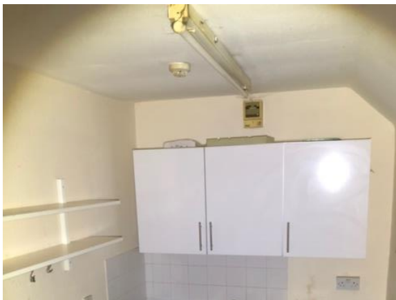
Photo 11: Upstairs kitchen – well-sealed.
